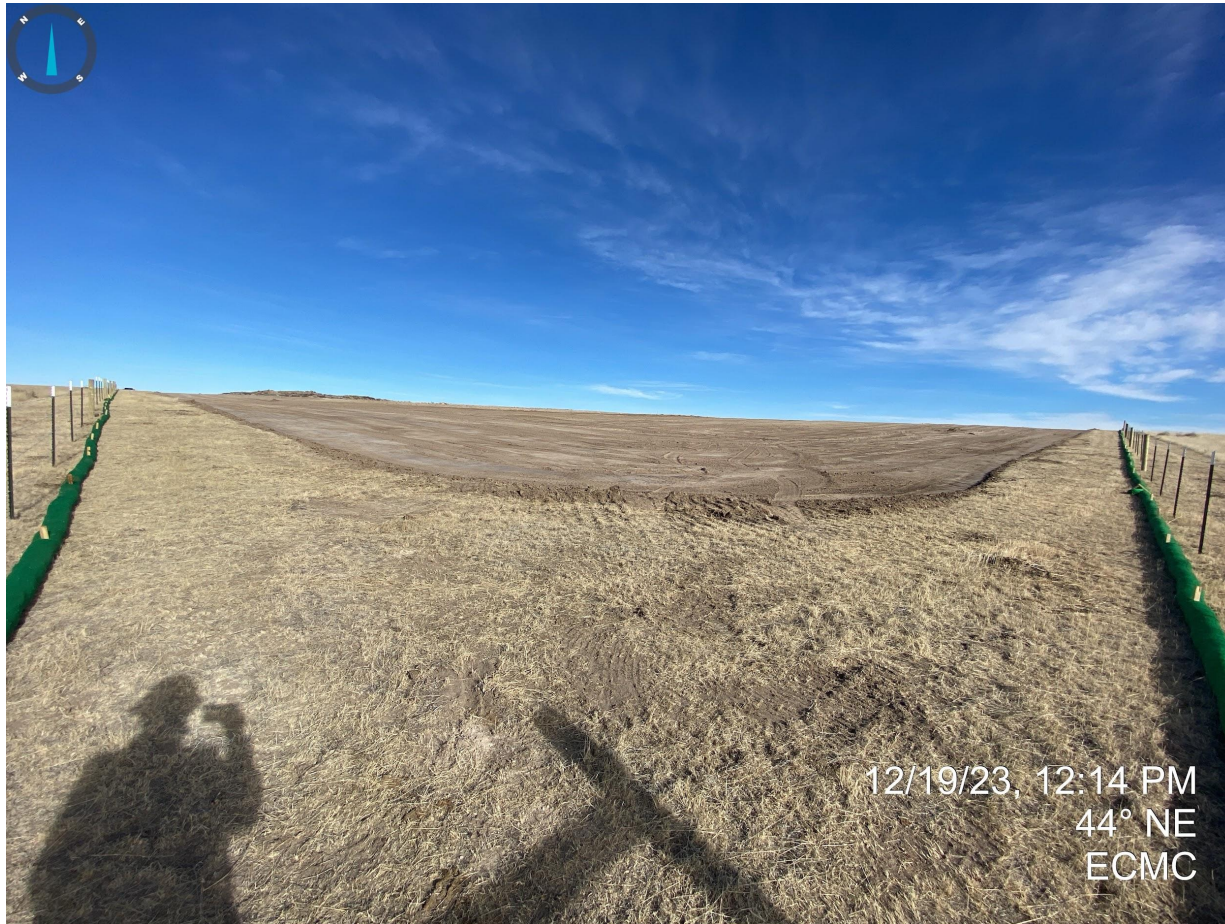
Photo 5. Taken from the southwest corner of the construction/disturbance area. It appears that topsoil salvage operations have commenced. The Operator shall ensure that all topsoil is salvaged per Rule 1002.b. A follow up inspection will be conducted at a later date to ensure topsoil salvage operations comply with the reclamation rules. Photo also illustrates temporary stormwater controls (filtrexx) installed around the entire perimeter of the location.
