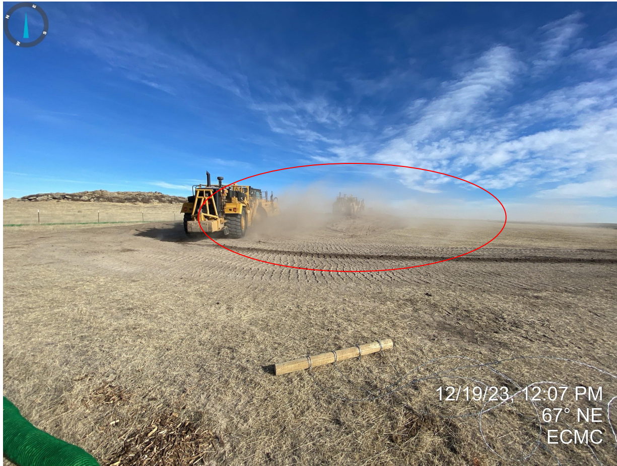
Photo 4. Taken from the location's entrance, facing northeast towards the topsoil stockpile. Photo illustrates that fugitive dust is occurring from topsoil salvage operations.
