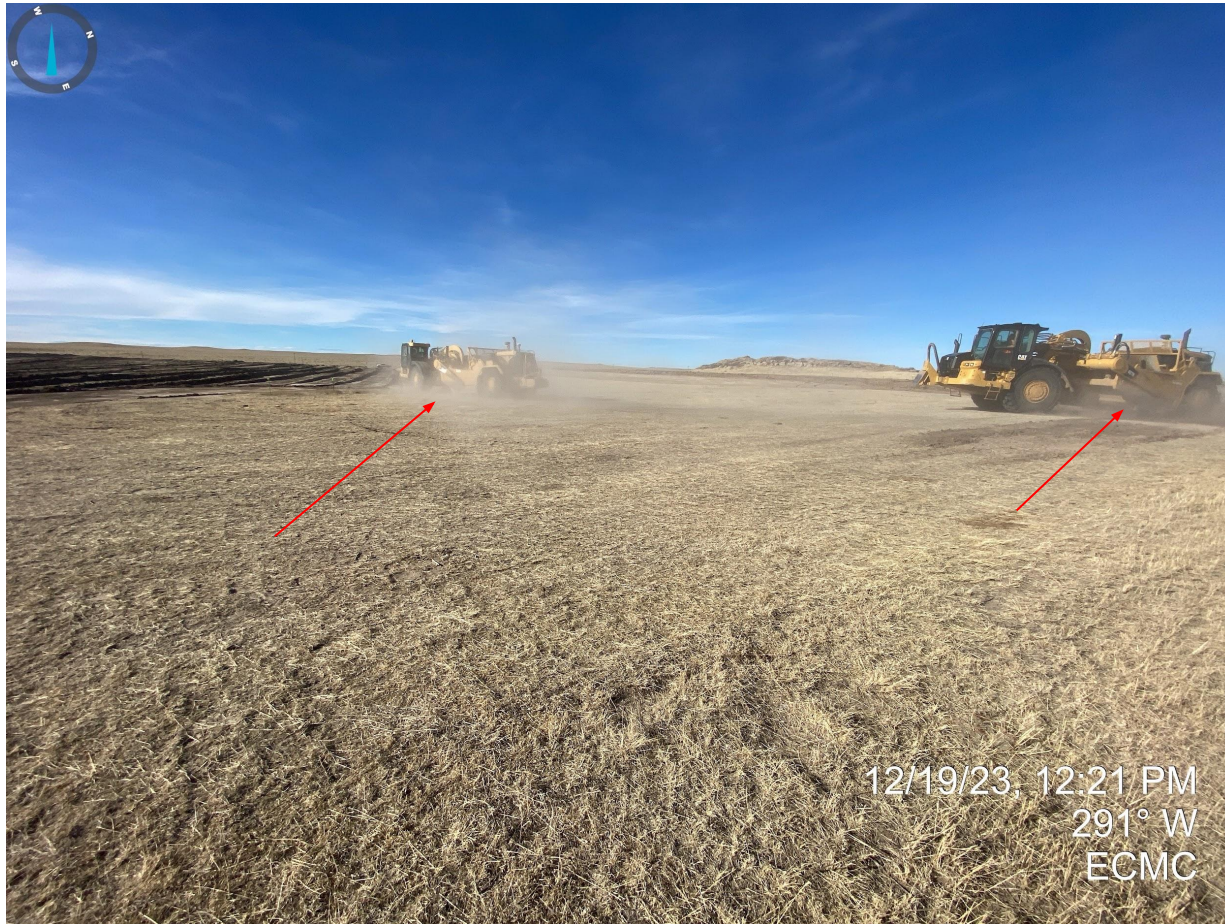
Photo 9. Taken near the northeast corner of the disturbance area. Photo illustrates that fugitive dust is occurring from topsoil salvage operations.
