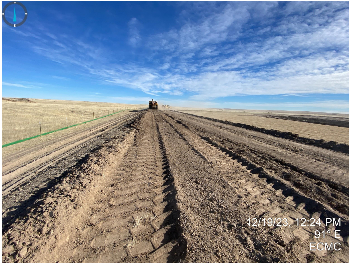
Photo 12. Taken from the center portion of the topsoil stockpile, facing east. Topsoil salvage operations are still ongoing at the time of this inspection. The Operator shall ensure that all stockpiled soils have adequate BMPs to prevent erosion degradation from wind and water.
