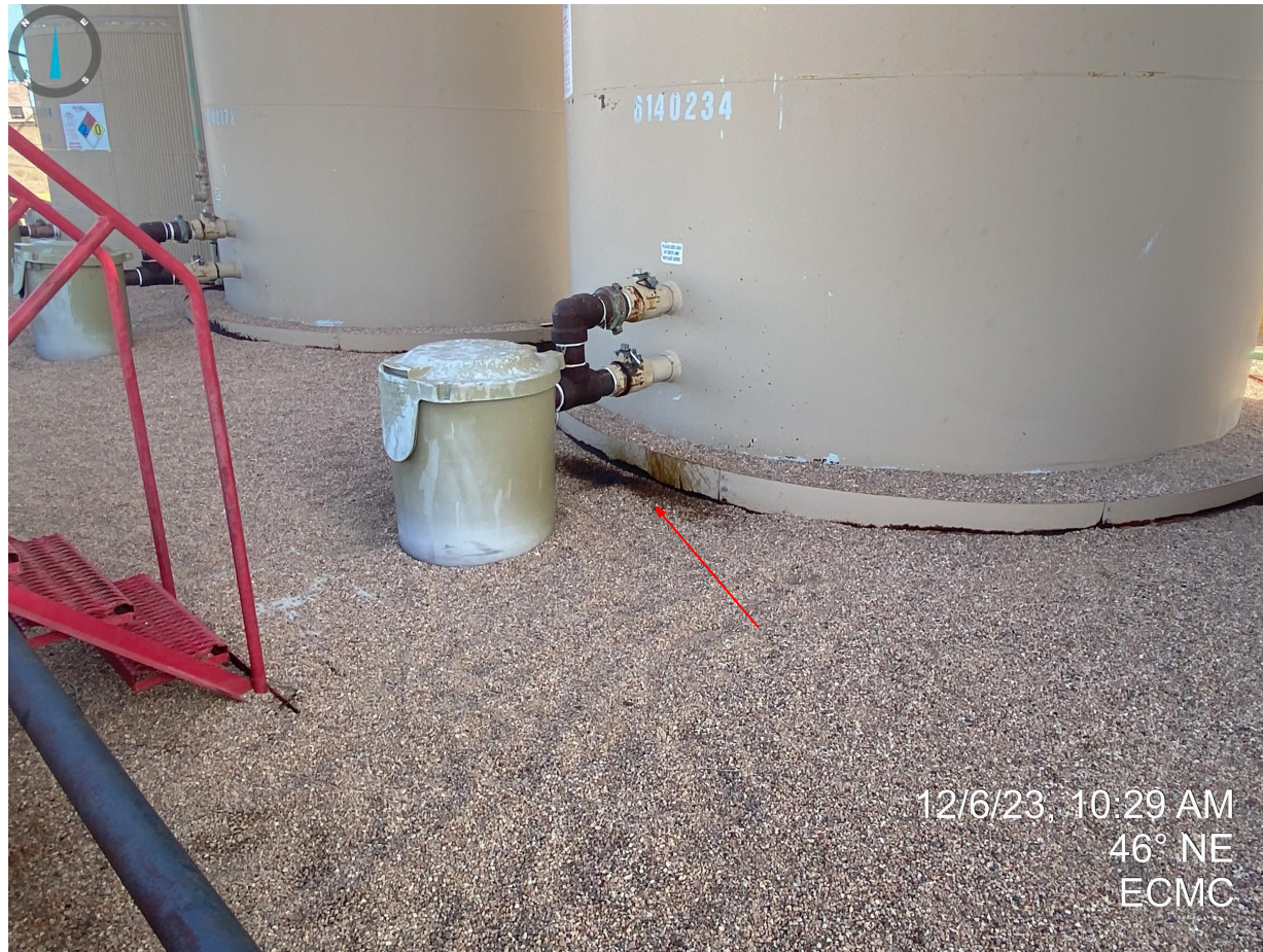
Photo 1. Stained soil observed near loadout line at tank battery.
