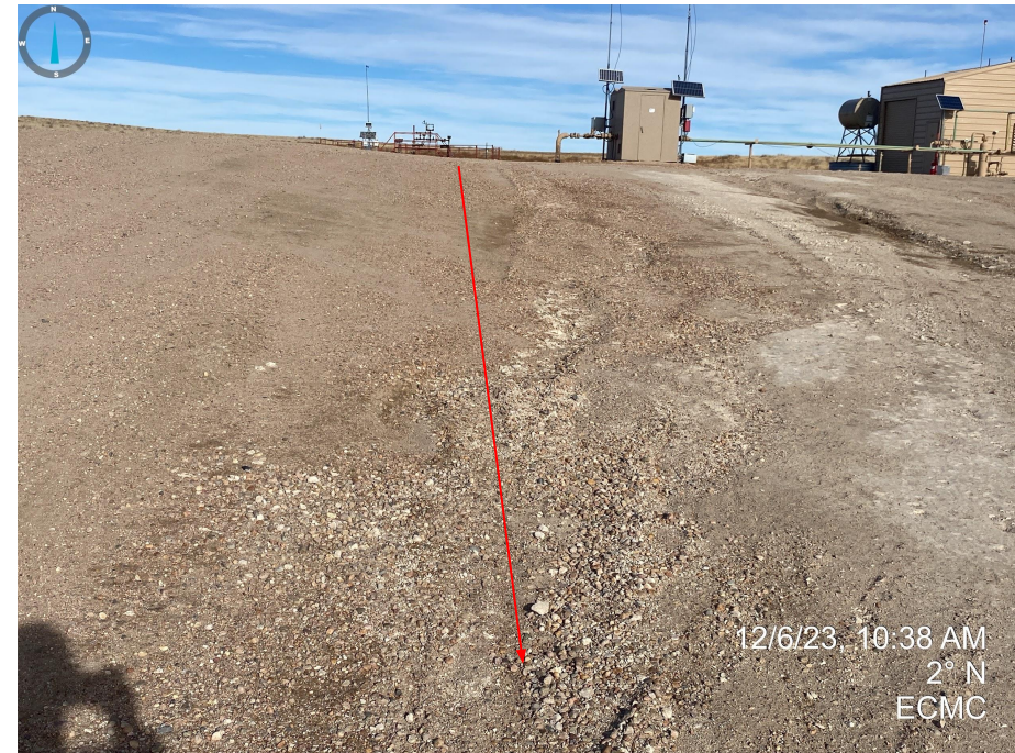
Photos 10 & 11. Erosion degradation (rilling) occurring within the center portion of the production areas.
