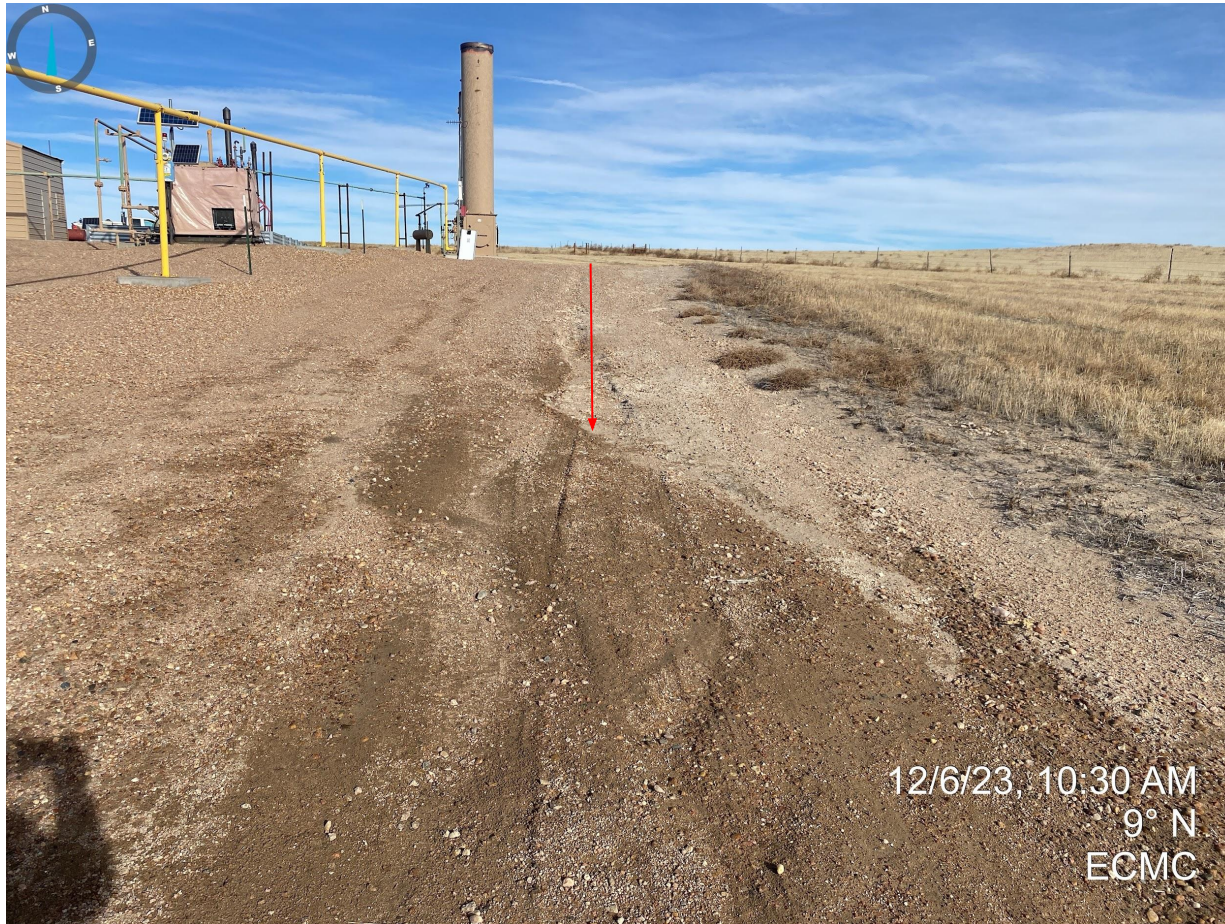
Photo 2. Erosion degradation (rilling) occurring on the eastern portion of the production areas.
