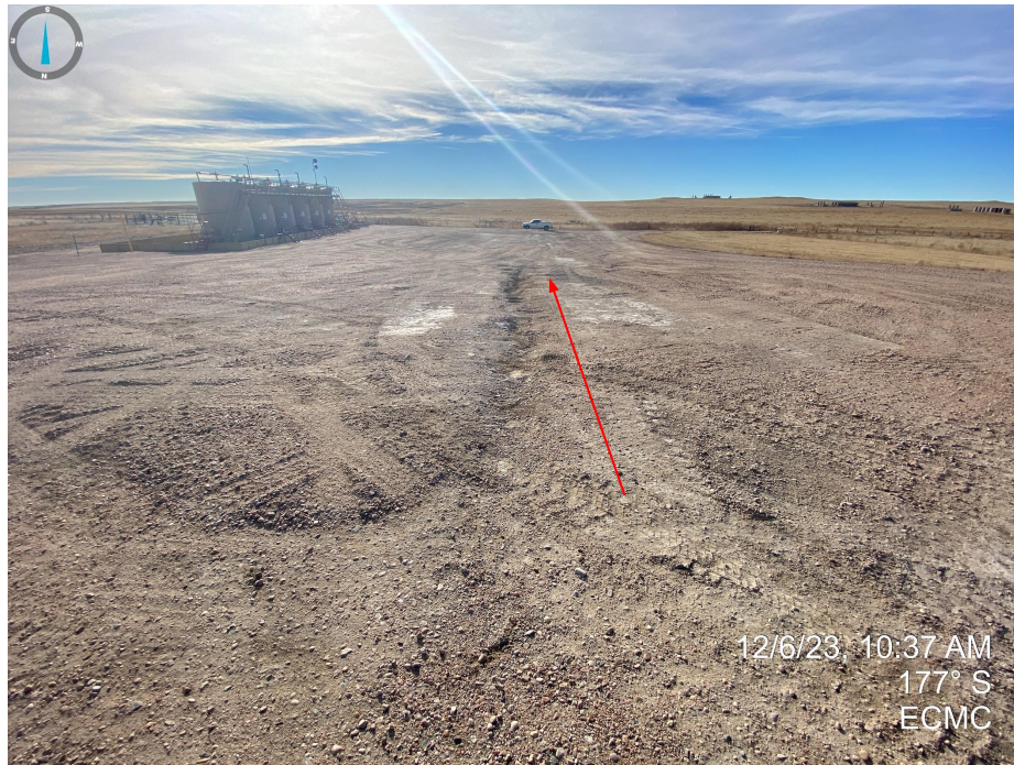
Photos 10 & 11. Erosion degradation (rilling) occurring within the center portion of the production areas.
