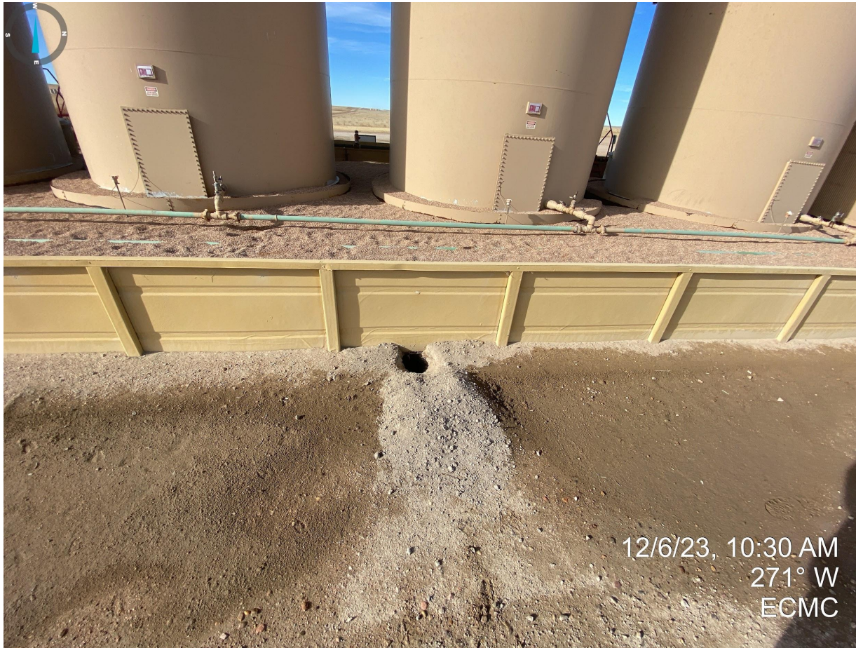
Photos 4-6. Animal burrows observed around the eastern and southern edges of the tank battery secondary containment.
