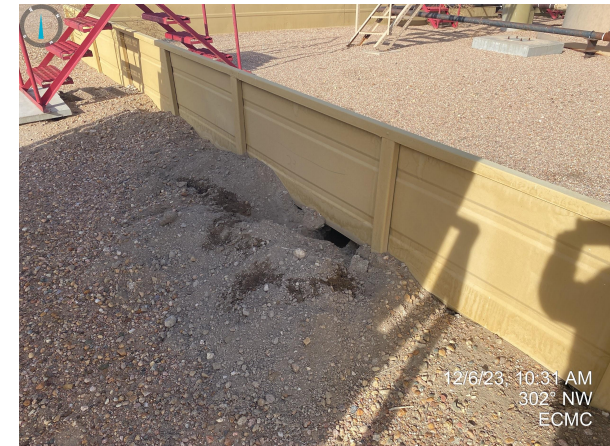
Photos 4-6. Animal burrows observed around the eastern and southern edges of the tank battery secondary containment.
