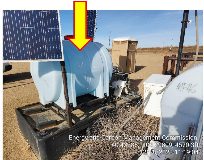
Photo 4 – MT 45 Missing Labels
