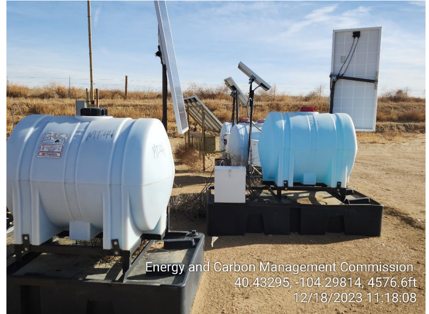
Photo 2 – Chemical (Methanol) Containers
