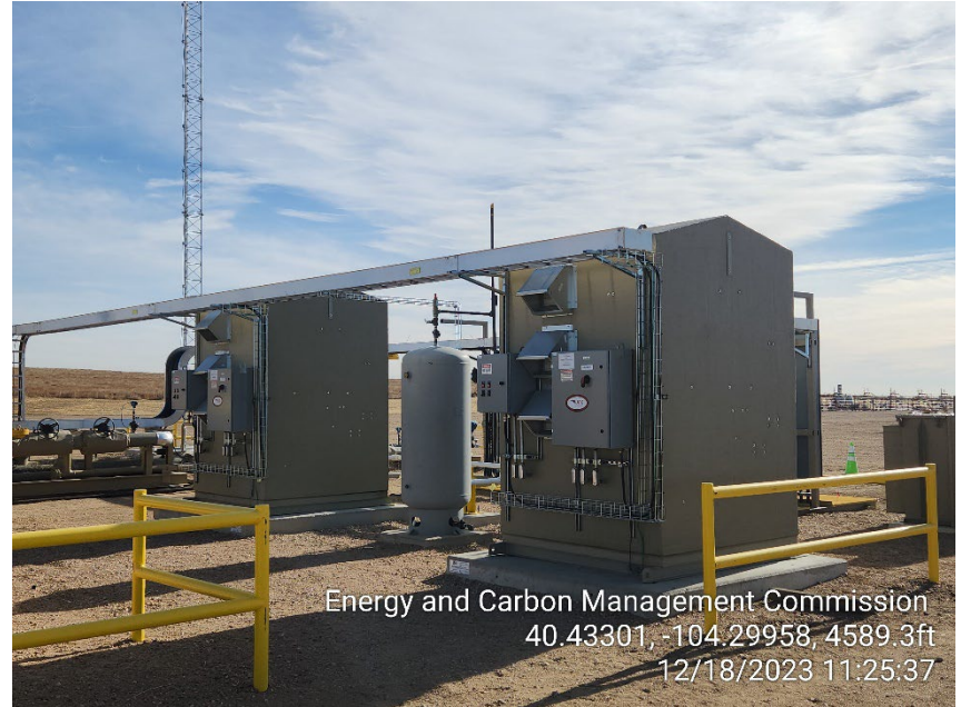
Photo 16 – Instrumental Air Units
