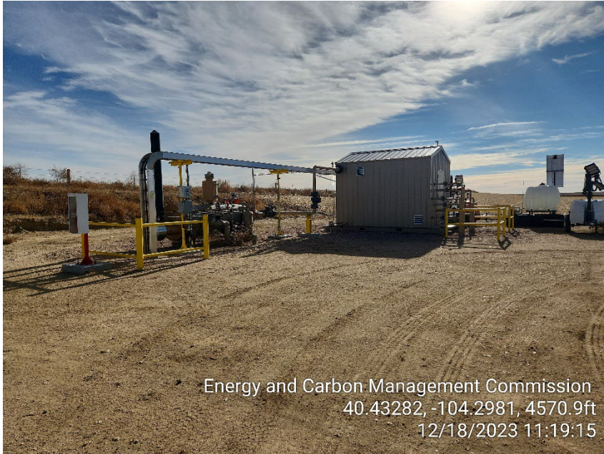
Photo 5 – South Gas Lift Injection Meter house and Line Heater
