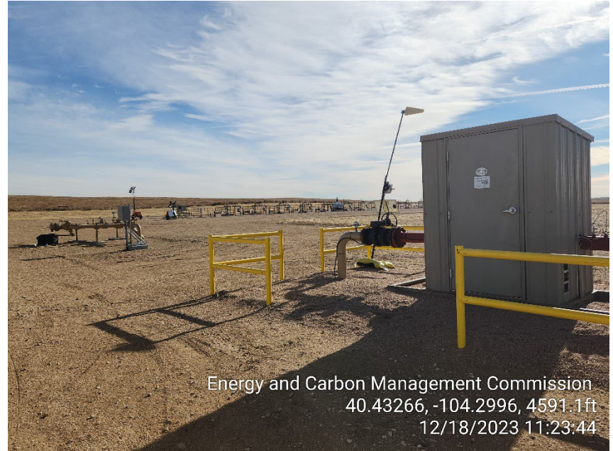
Photo 10 – Gas Meter House and Pig Line
