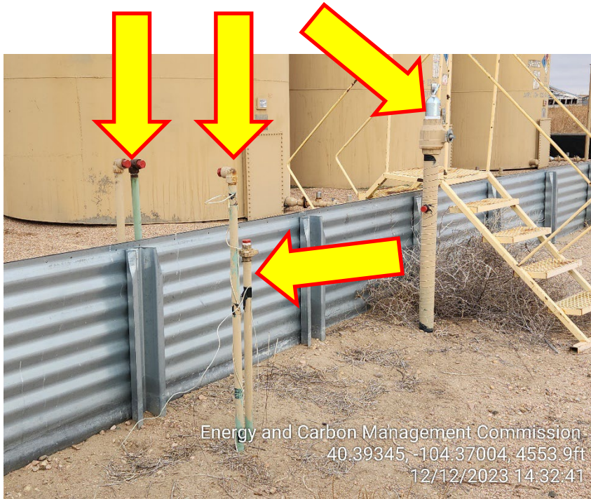
Photo 11 – Unmarked Risers at Tanks
