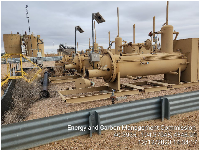
Photo 17 – Separator is open to Atmosphere. Unused Meter Tube, Pipe, Fittings and Heat Stack. Unmarked Risers. Tumbleweed Debris
