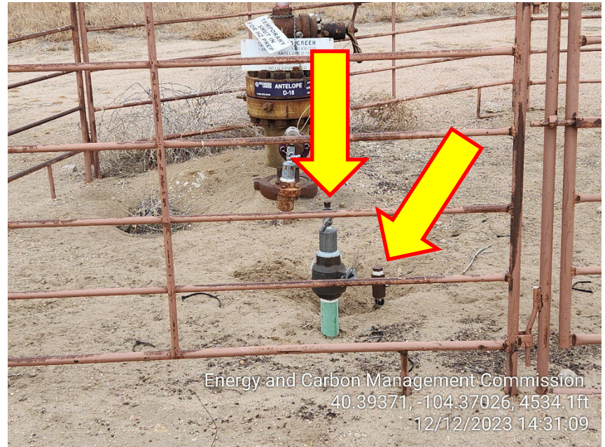
Photo 4 – Unmarked Risers
