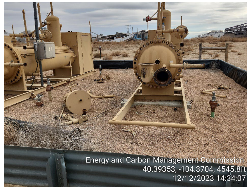
Photo 16 – Separator is open to Atmosphere. Unused Meter Tube, Pipe, Fittings and Heat Stack. Unmarked Risers
