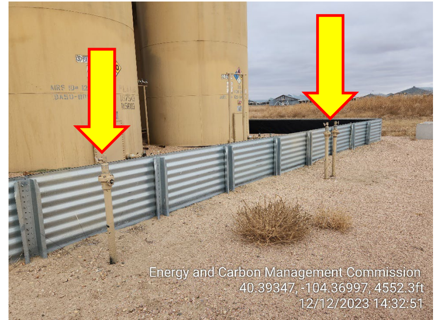
Photo 12 – Unmarked Risers Tank
