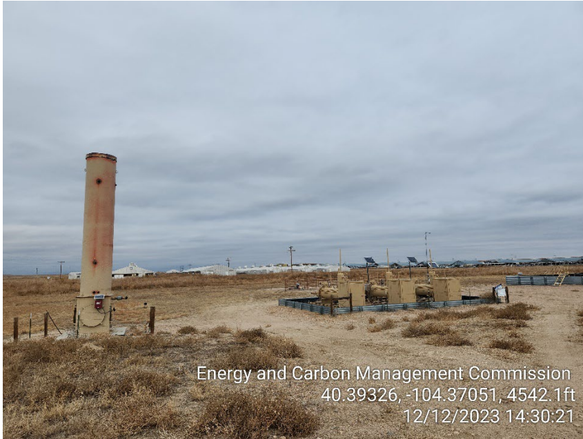
Photo 1 – Separators and ECD
