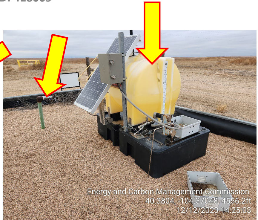
Photo 8 – Unmarked Riser and Unused Chemical Container
