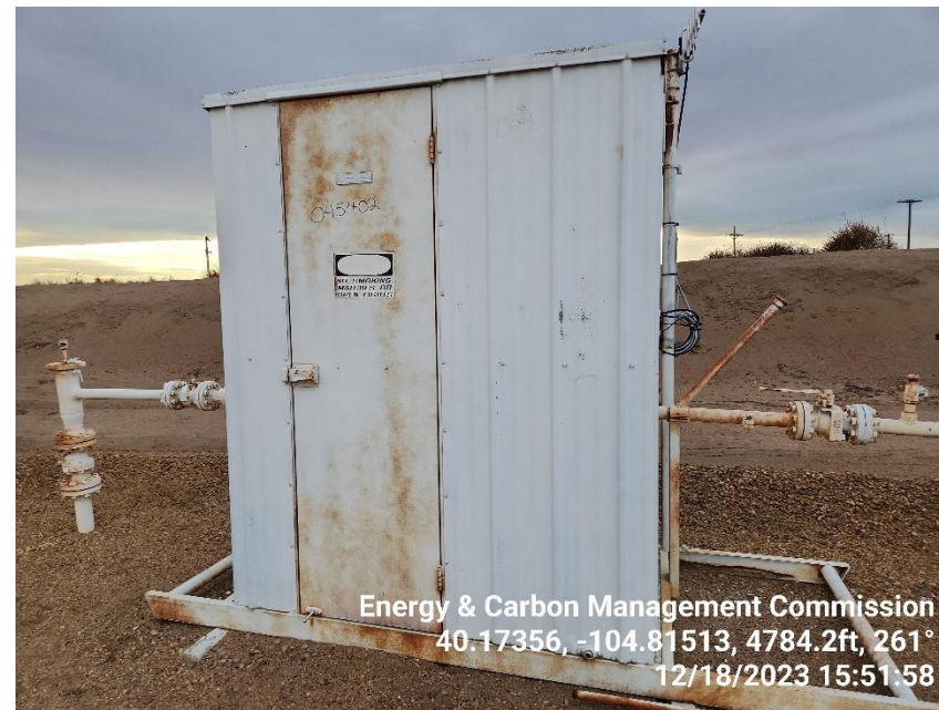
Photo 10 Gas Meter Run.
