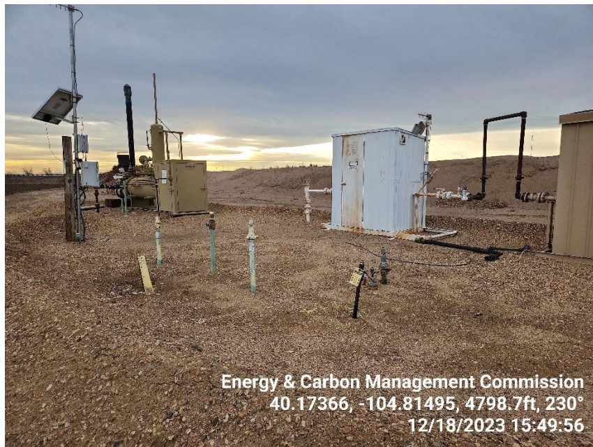
Photo 7 HHS, Gas Meter Run x 2, tagged out flow lines and trash.
