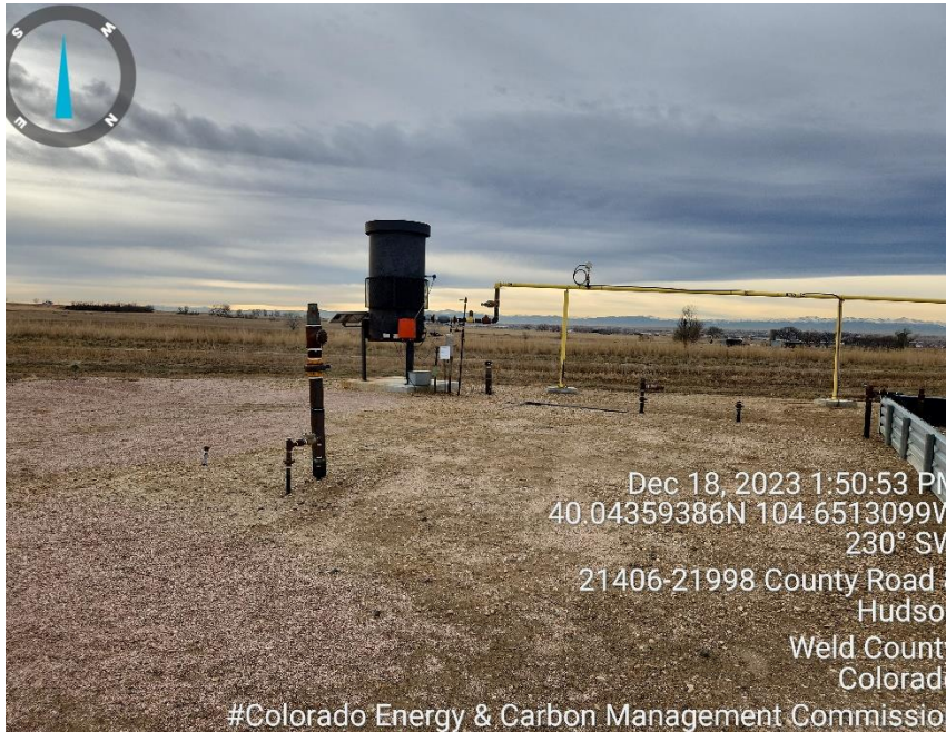
Photo 5 Unused/unmarked and not LOTO risers
