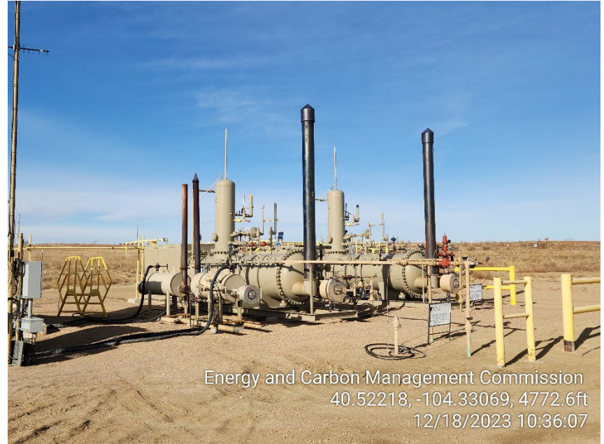
Photo 14 – Glycol Units and Separators
