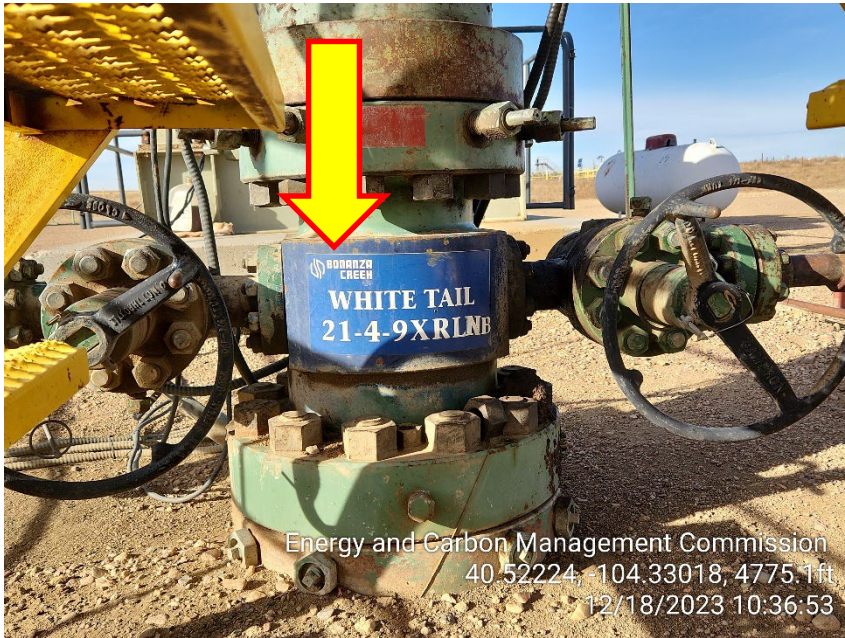
Photo 5 – Wellhead Sign does not reflect current Operator
