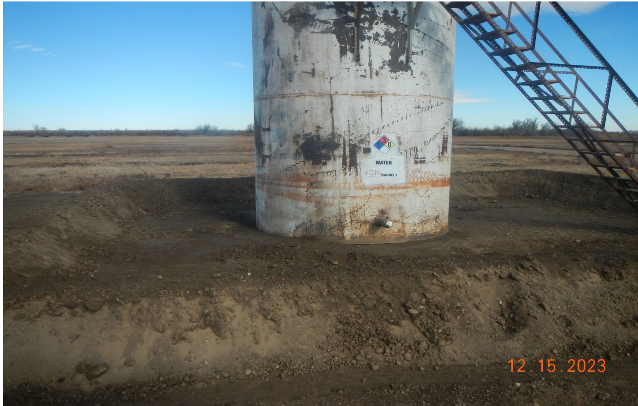
Photo 2. Facing toward the tank which is labeled as water. It appears stained soil was removed. A berm was constructed around the tank however bermed soils need to be compacted.
