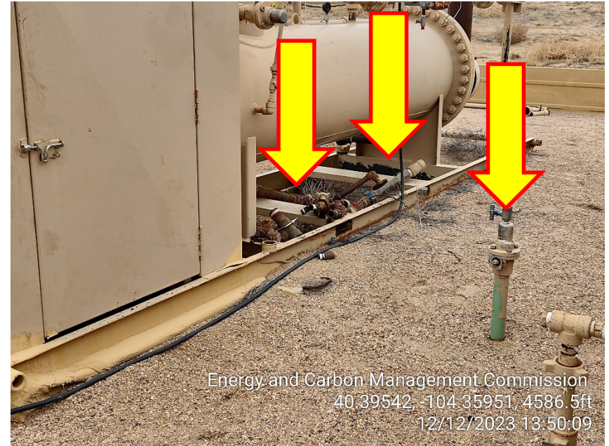
Photo 6 – Unmarked OOSLAT 2" Riser and unused Parts and Piping
