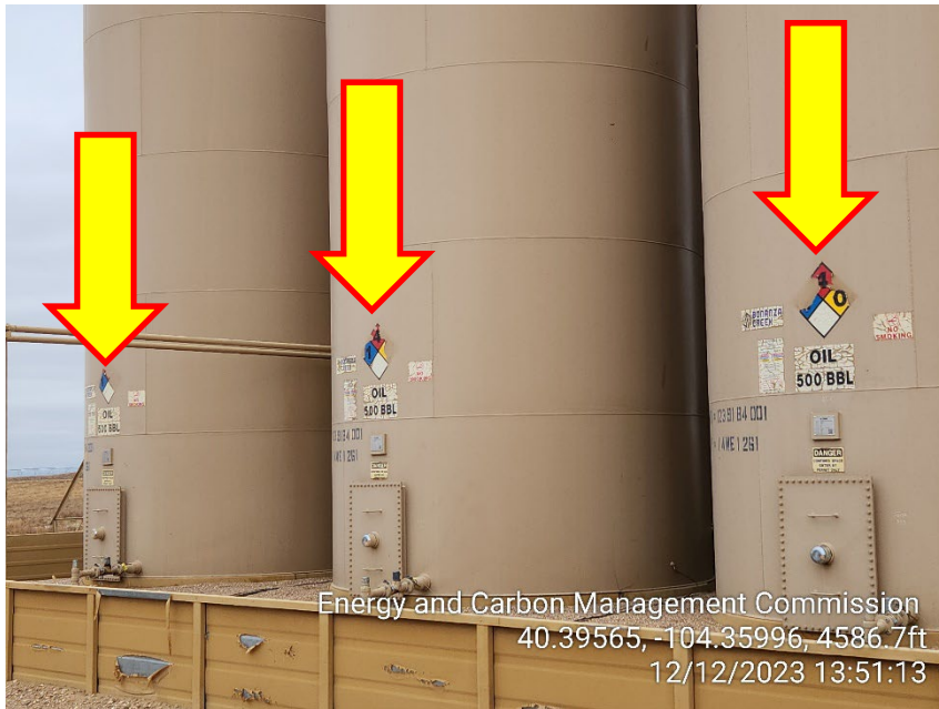
Photo 9 – NFPA Labels on West Side Tanks
