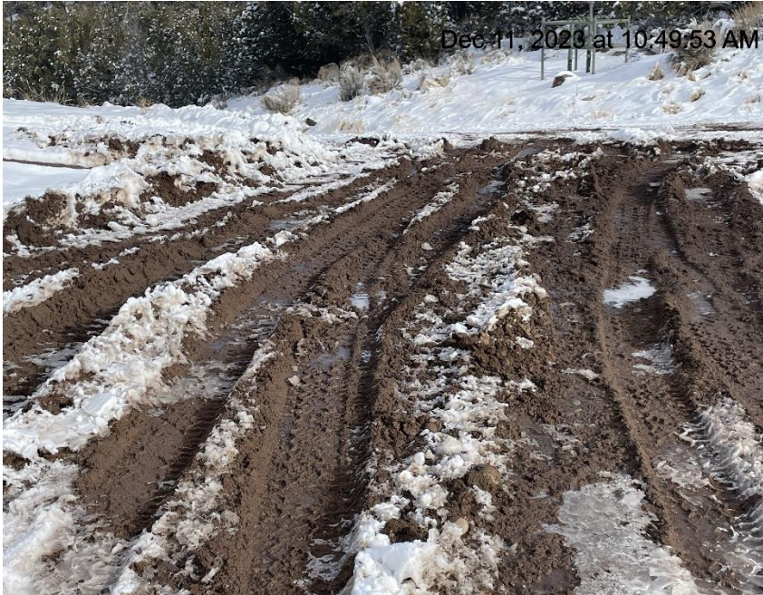
Photo # 9117 Lack of stabilization/compaction/insufficient BMP's on lease road near entrance to location
