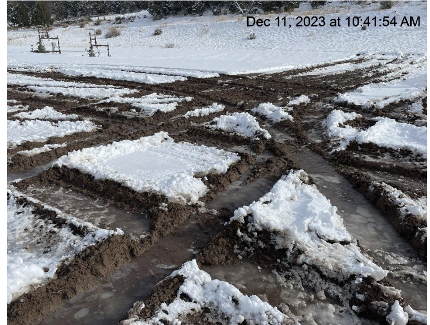
Photo # 9106 Lack of stabilization/compaction/insufficient BMP's on location
