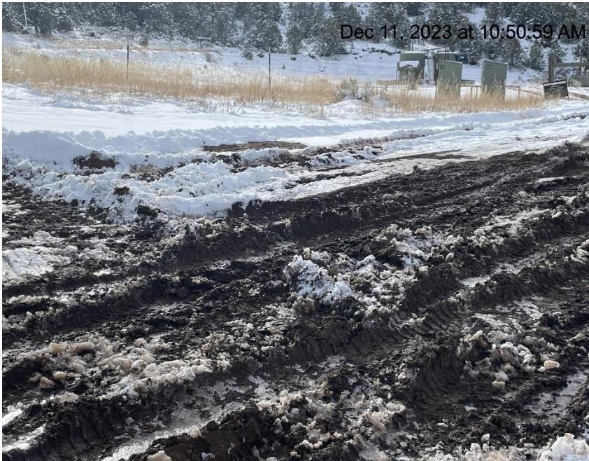
Photo # 9121 Lack of stabilization/compaction/insufficient BMP's on lease road near entrance to location
