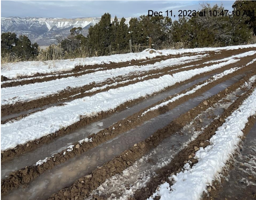
Photo # 9111 Lack of stabilization/compaction/insufficient BMP's on location
