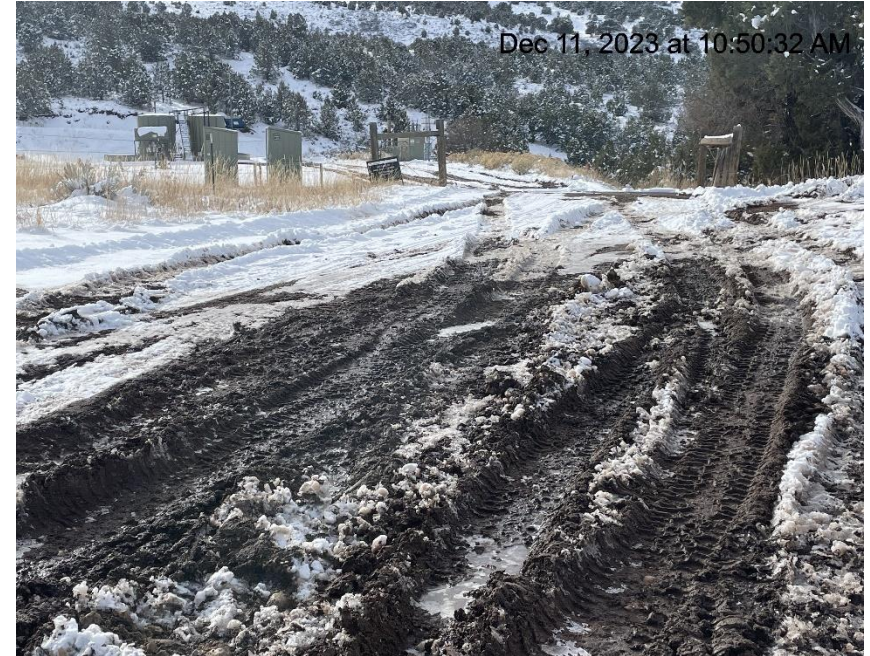
Photo # 9120 Lack of stabilization/compaction/insufficient BMP's on lease road near entrance to location
