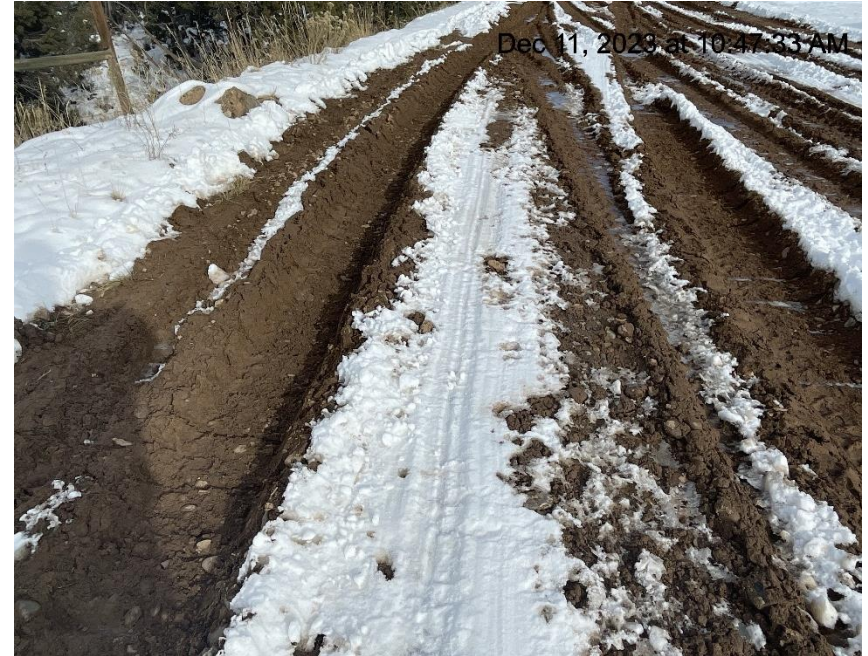
Photo # 9112 Lack of stabilization/compaction/insufficient BMP's on location
