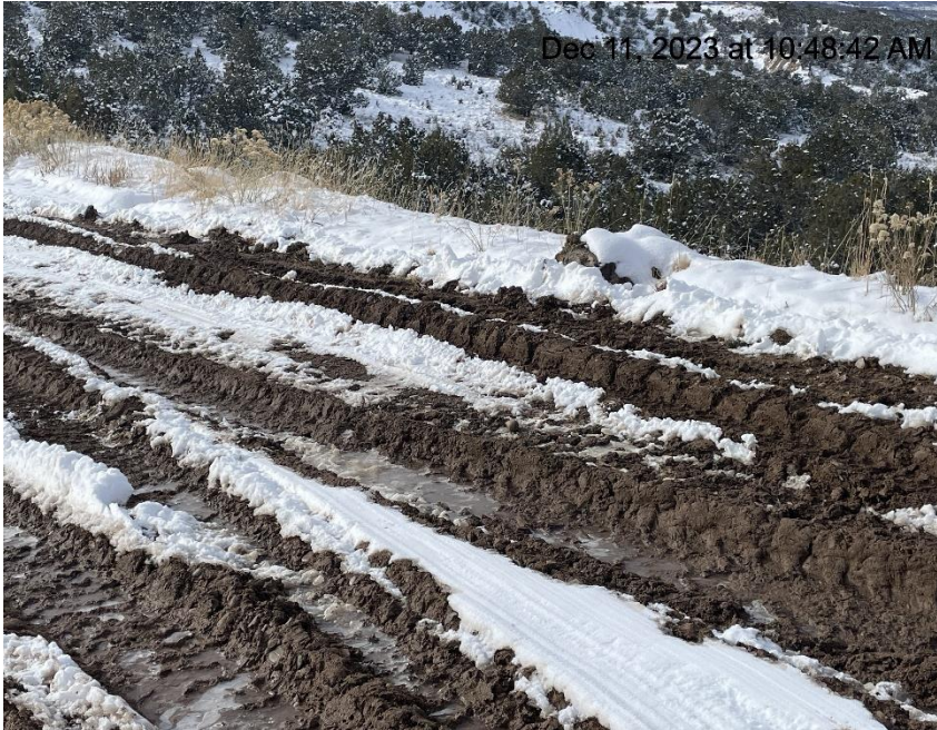
Photo # 9115 Lack of stabilization/compaction/insufficient BMP's on location
