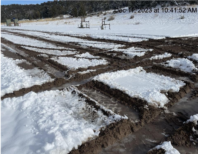
Photo # 9105 Lack of stabilization/compaction/insufficient BMP's on location
