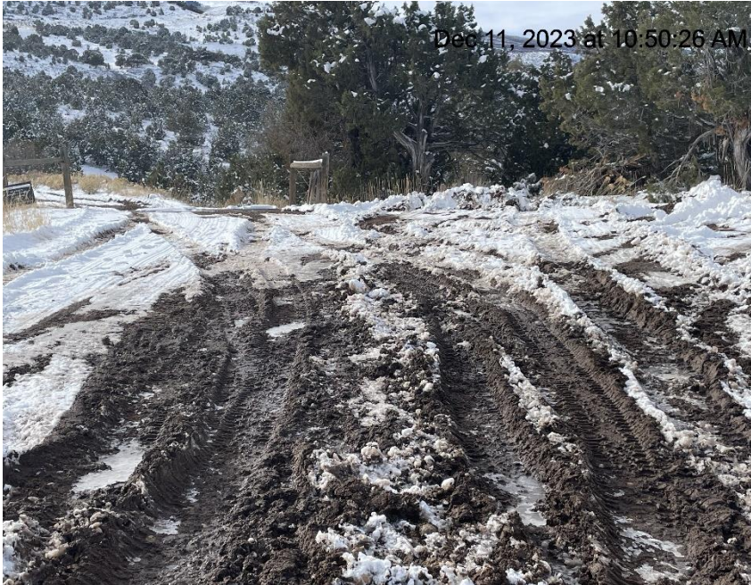
Photo # 9119 Lack of stabilization/compaction/insufficient BMP's on lease road near entrance to location
