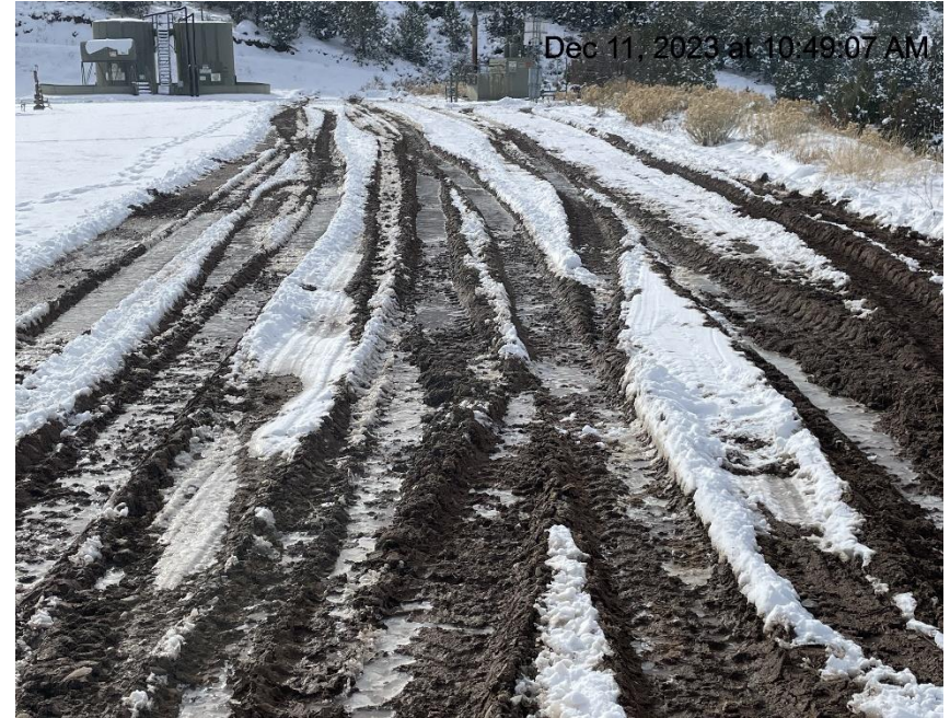
Photo # 9114 Lack of stabilization/compaction/insufficient BMP's on location
