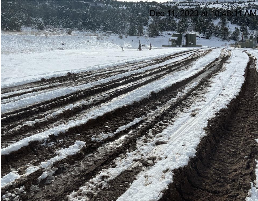
Photo # 9113 Lack of stabilization/compaction/insufficient BMP's on location
