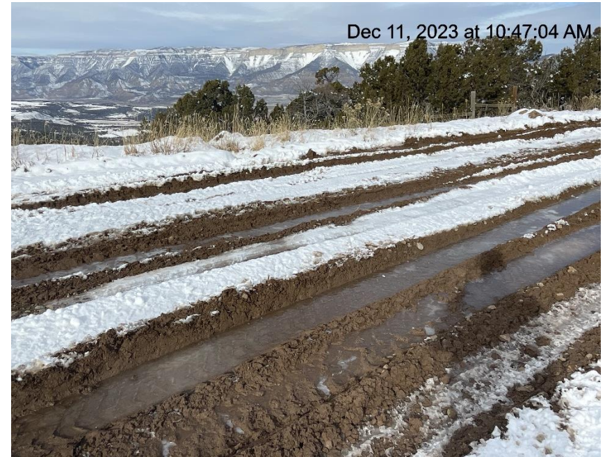
Photo # 9110 Lack of stabilization/compaction/insufficient BMP's on location
