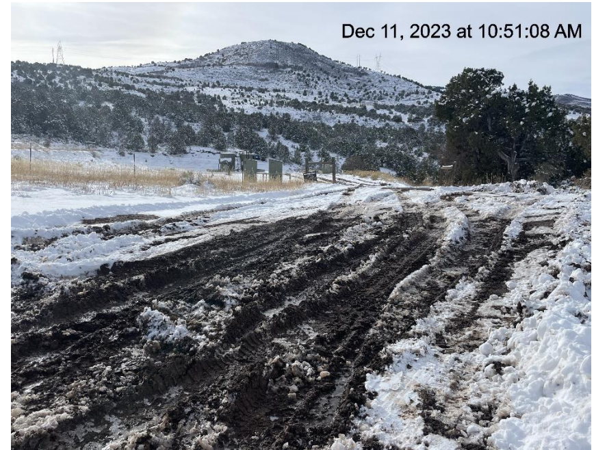
Photo # 9122 Lack of stabilization/compaction/insufficient BMP's on lease road near entrance to location
