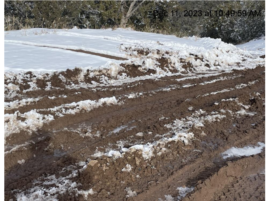
Photo # 9118 Lack of stabilization/compaction/insufficient BMP's on lease road near entrance to location
