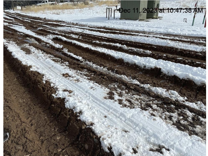
Photo # 9116 Lack of stabilization/compaction/insufficient BMP's on location
