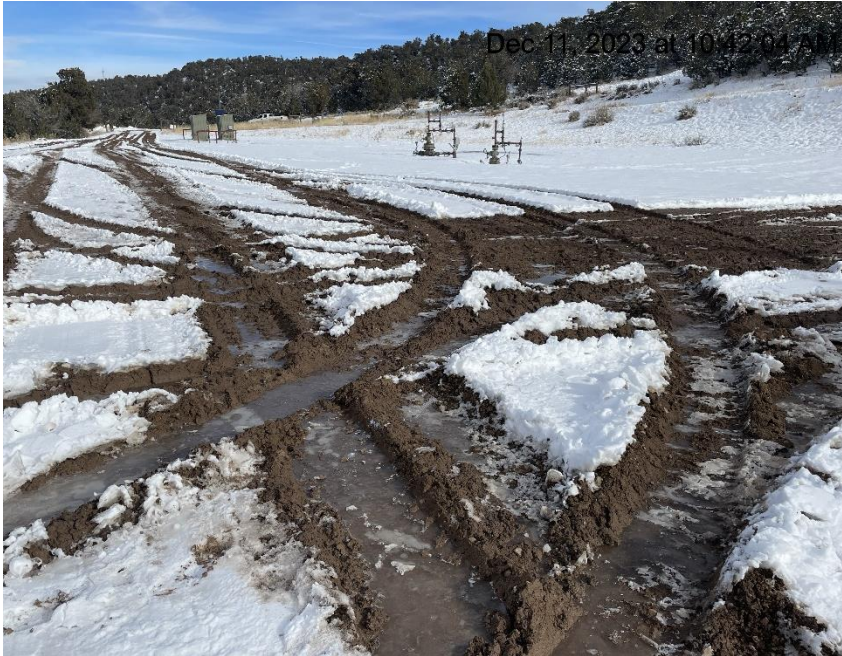
Photo # 9107 Lack of stabilization/compaction/insufficient BMP's on location
