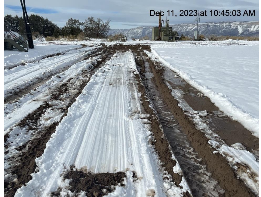
Photo # 9108 Lack of stabilization/compaction/insufficient BMP's on location
