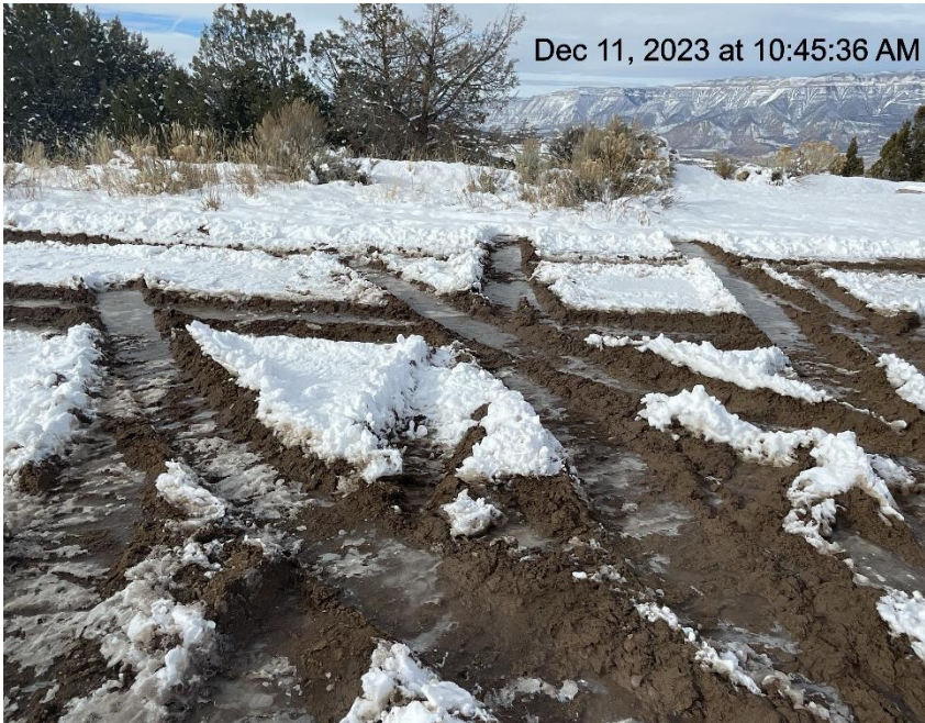
Photo # 9109 Lack of stabilization/compaction/insufficient BMP's on location
