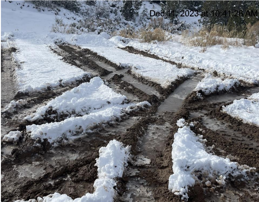
Photo # 9103 Lack of stabilization/compaction/insufficient BMP's on location
