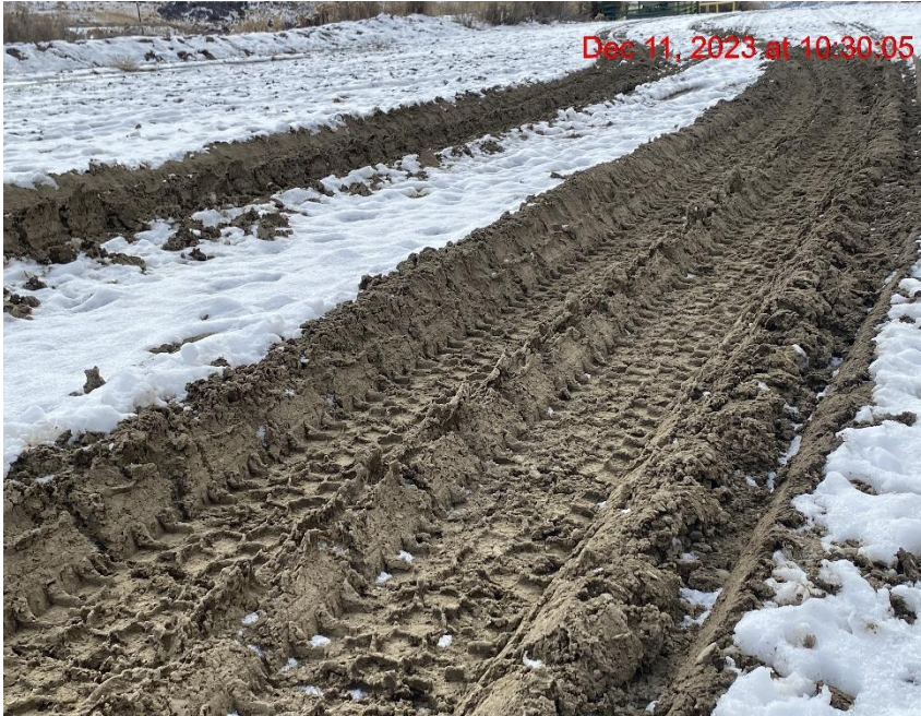
Lack of Stabilization – Photo #08116
