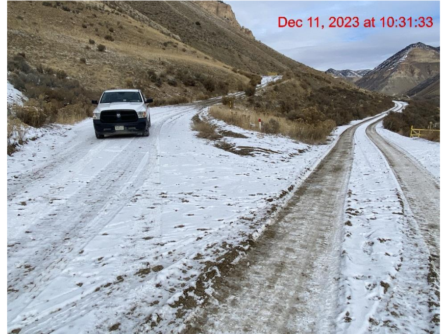
Insufficient Vehicle Tracking BMPs at Location Entrance/Exit – Photo #08117
