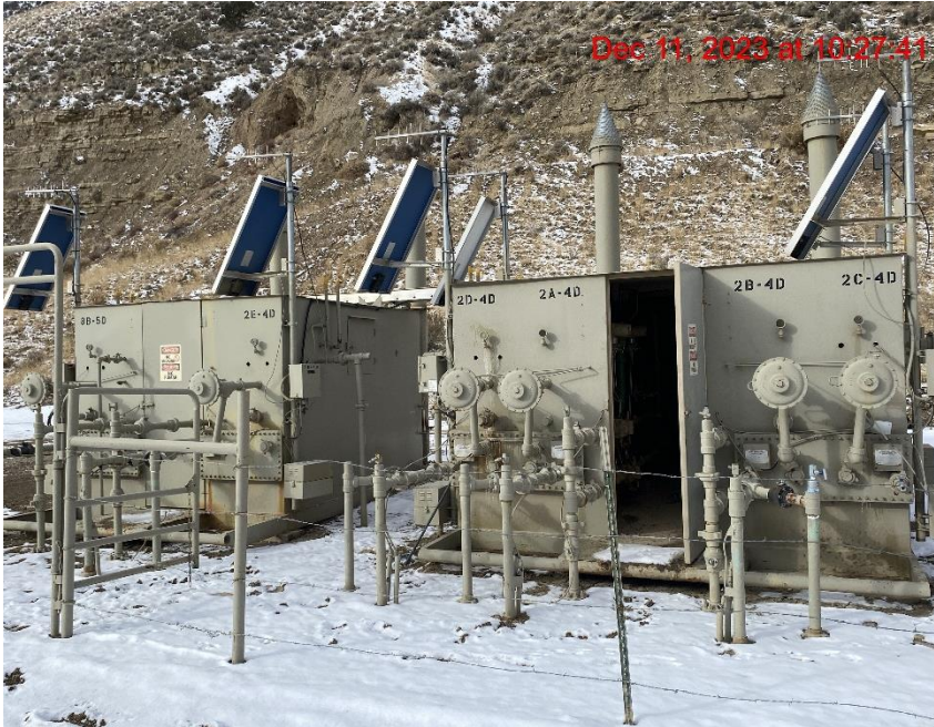
Separators/Unsecured Door – Photo #08110
