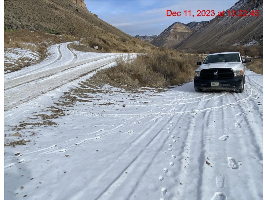
Insufficient Vehicle Tracking BMPs at Location Entrance/Exit – Photo #08103
