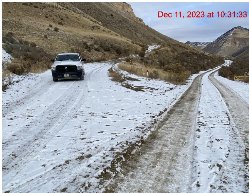
Insufficient Vehicle Tracking BMPs at Location Entrance/Exit – Photo #08117
