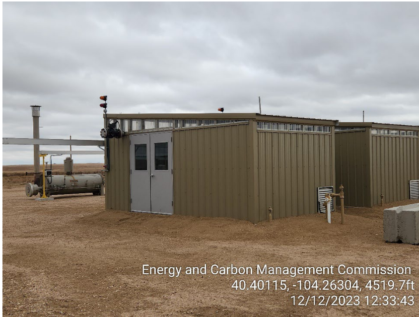
Photo 3 – Gas Lift Injection Meters and Line Heater
