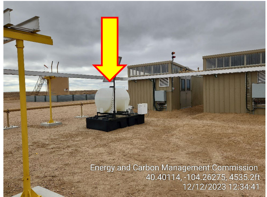
Photo 4 – Chemical Container missing Labels
