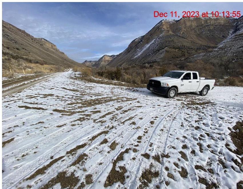
Insufficient Vehicle Tracking BMPs at Location Entrance/Exit – Photo #08090
