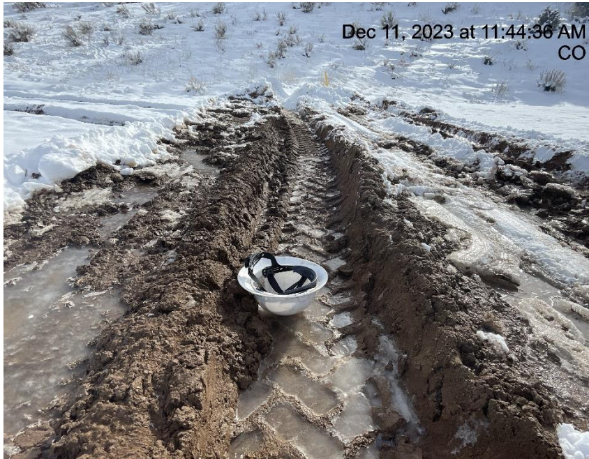
Photo # 9277 Lack of stabilization/compaction/insufficient BMP's
