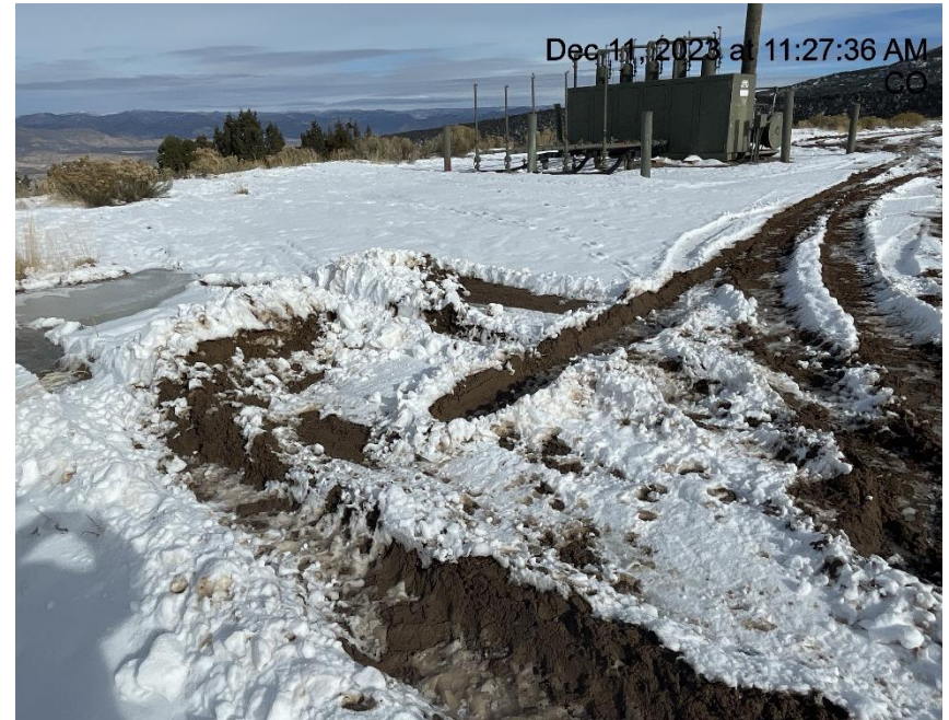
Photo # 9270 Lack of stabilization/compaction/insufficient BMP's
