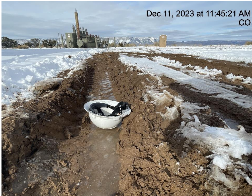
Photo # 9279 Lack of stabilization/compaction/insufficient BMP's
