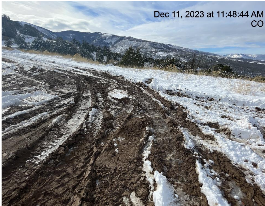
Photo # 9283 Lack of stabilization/compaction/insufficient BMP's
