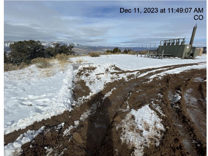
Photo # 9286 Lack of stabilization/compaction/insufficient BMP's
