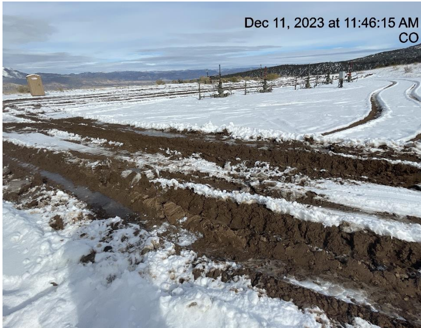
Photo # 9281 Lack of stabilization/compaction/insufficient BMP's
