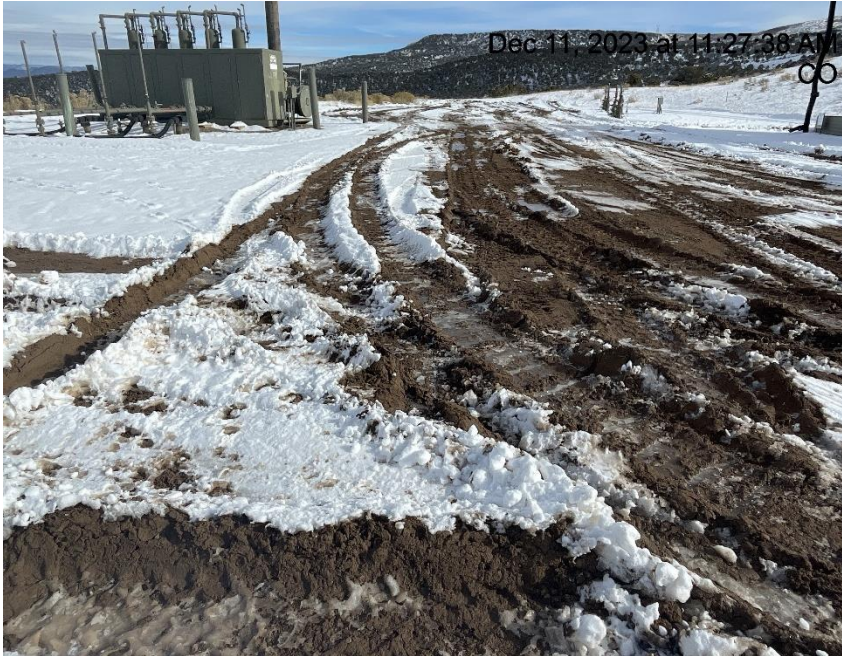
Photo # 9271 Lack of stabilization/compaction/insufficient BMP's
