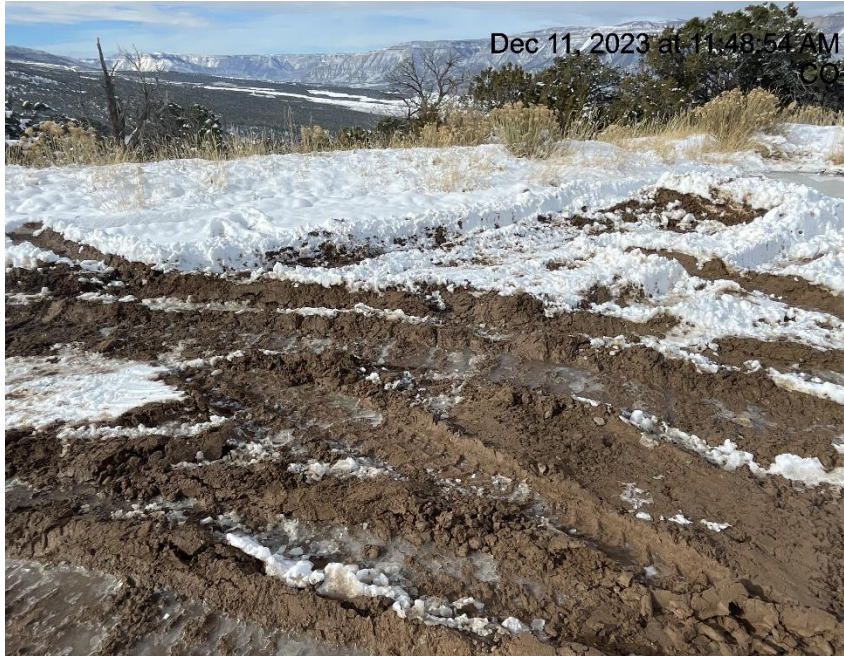
Photo # 9285 Lack of stabilization/compaction/insufficient BMP's
