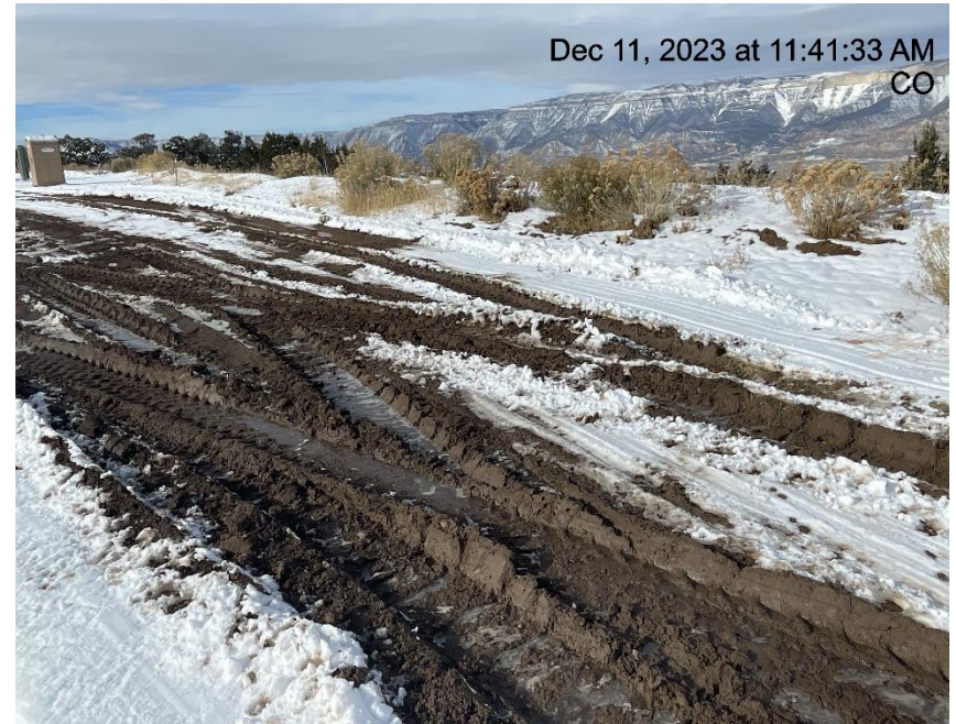
Photo # 9274 Lack of stabilization/compaction/insufficient BMP's
