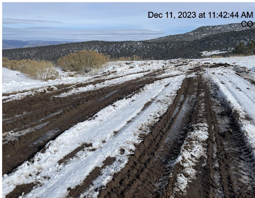
Photo # 9275 Lack of stabilization/compaction/insufficient BMP's
