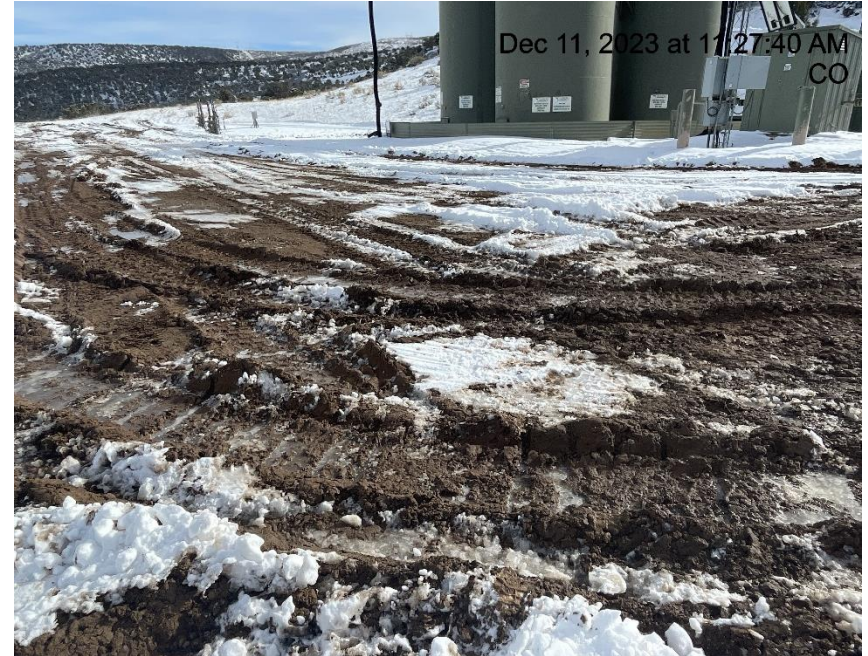
Photo # 9272 Lack of stabilization/compaction/insufficient BMP's
