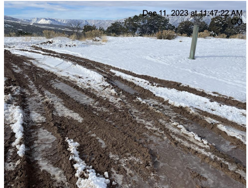
Photo # 9282 Lack of stabilization/compaction/insufficient BMP's
