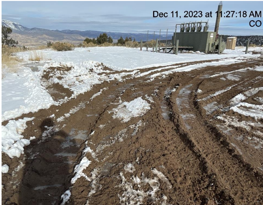
Photo # 9269 Lack of stabilization/compaction/insufficient BMP's
