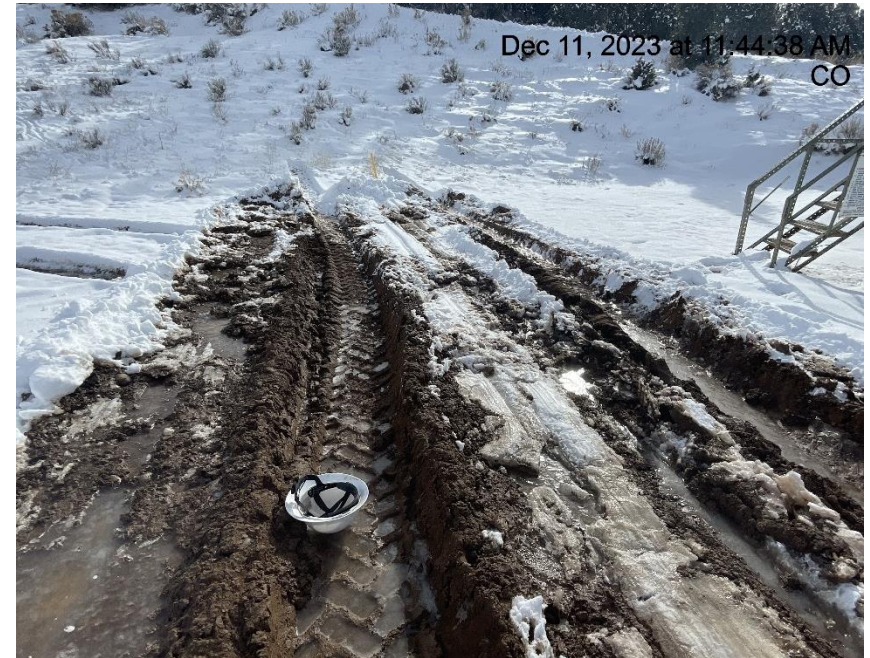
Photo # 9278 Lack of stabilization/compaction/insufficient BMP's
