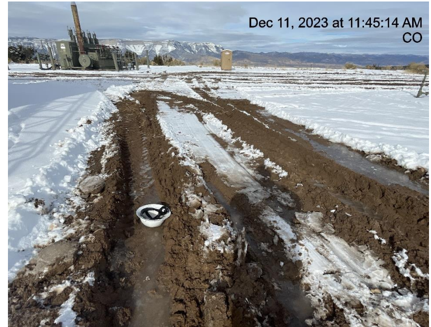
Photo # 9280 Lack of stabilization/compaction/insufficient BMP's
