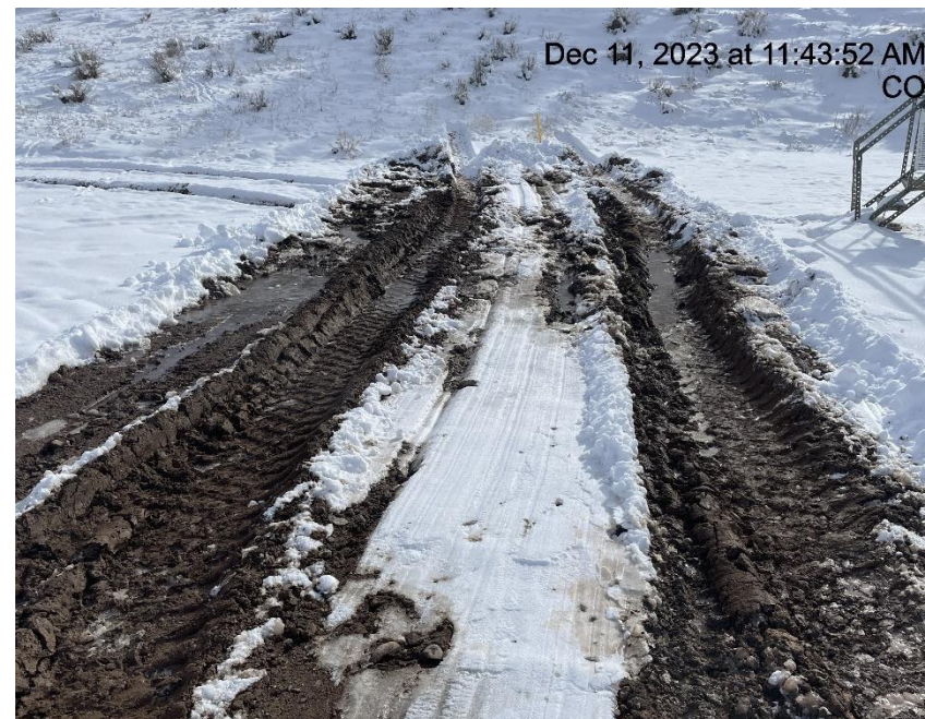
Photo # 9276 Lack of stabilization/compaction/insufficient BMP's
