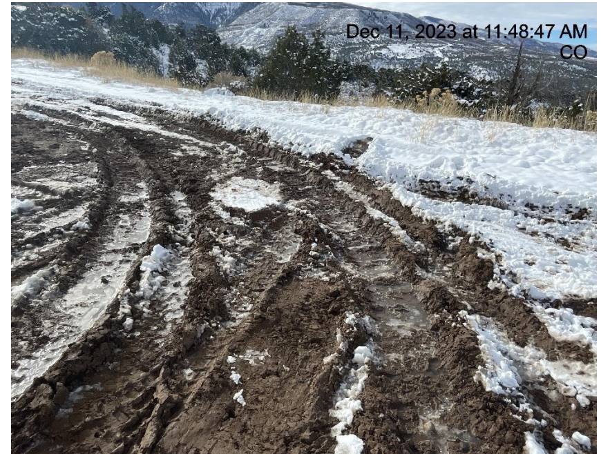
Photo # 9284 Lack of stabilization/compaction/insufficient BMP's
