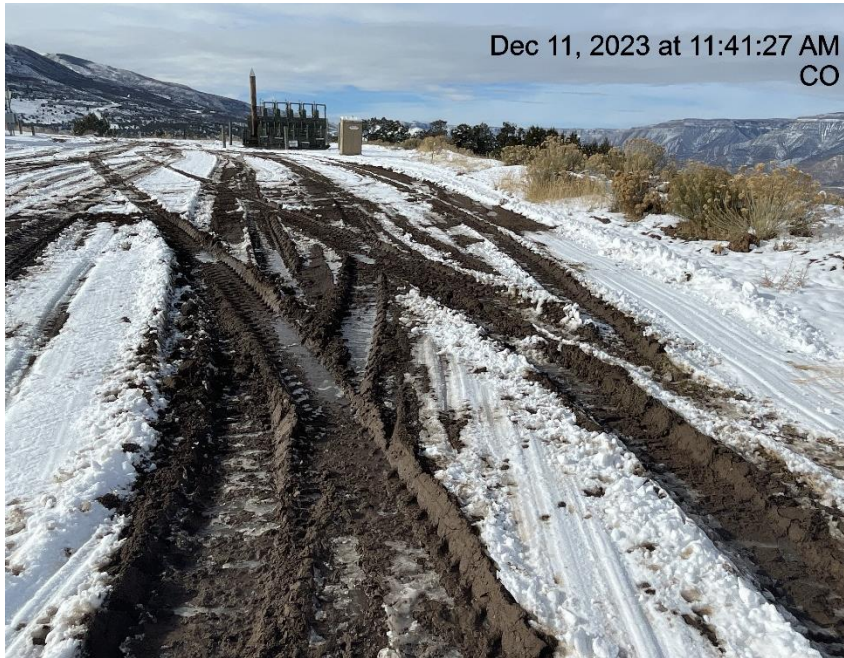
Photo # 9273 Lack of stabilization/compaction/insufficient BMP's
