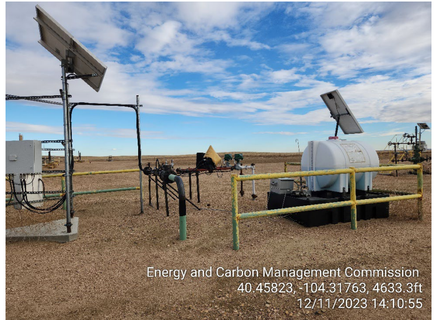
Photo 2 – Gas Lift Injection Meters
