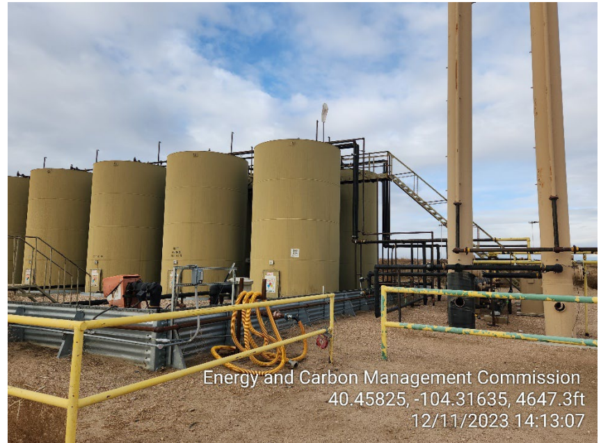
Photo 8 – Tank Battery and VRTs
