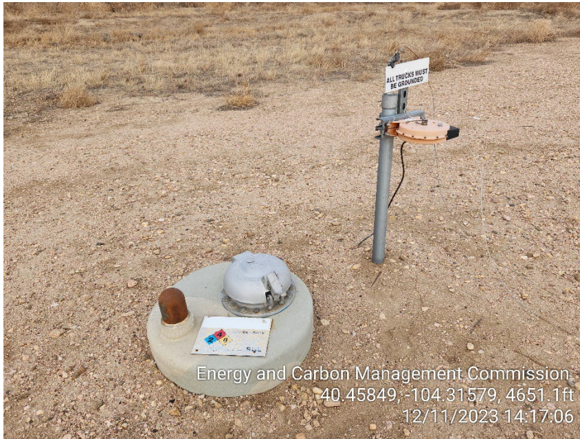
Photo 17 – Condensate Vault at Flare
