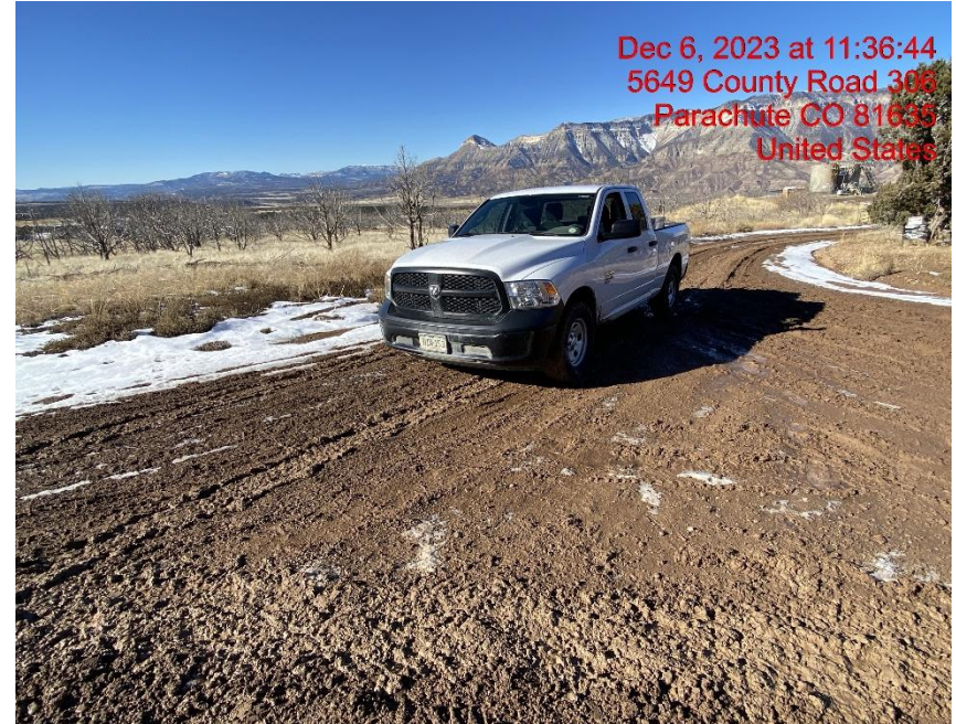
Insufficient Vehicle Tracking BMPs at Location Entrance/Exit – Photo #08009
