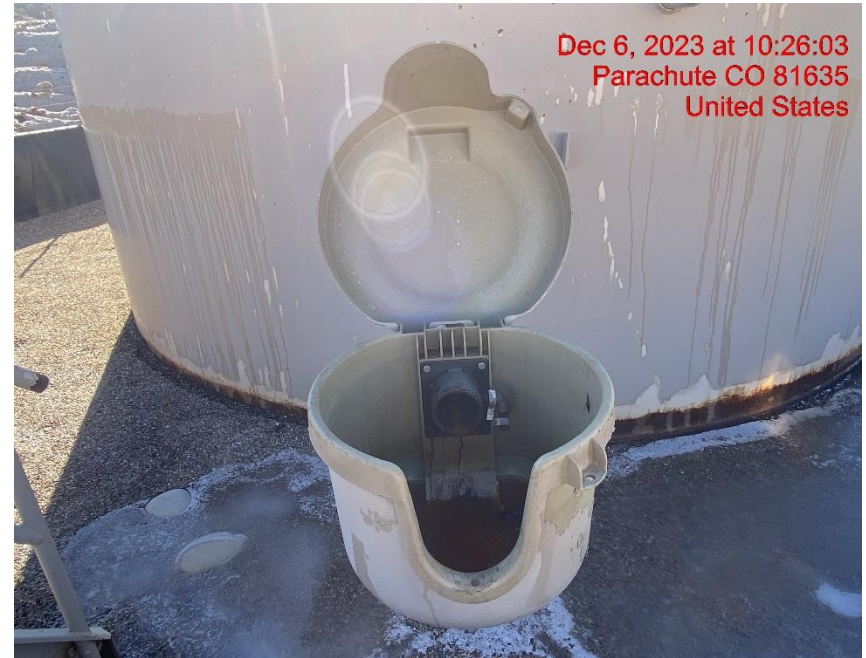
Open-Ended Load Line – Photo #07972
