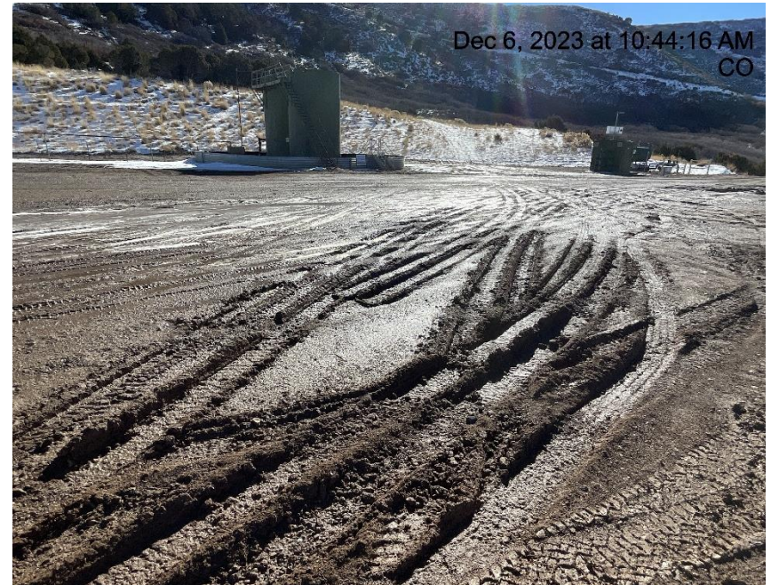
Photo # 8626 Lack of stabilization/compaction/insufficient BMP's
