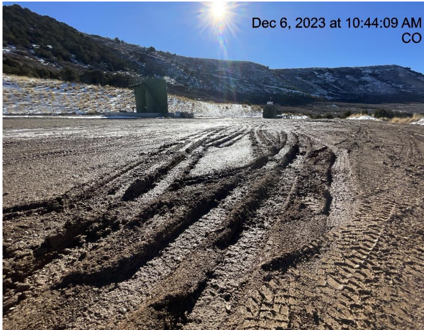
Photo # 8625 Lack of stabilization/compaction/insufficient BMP's
