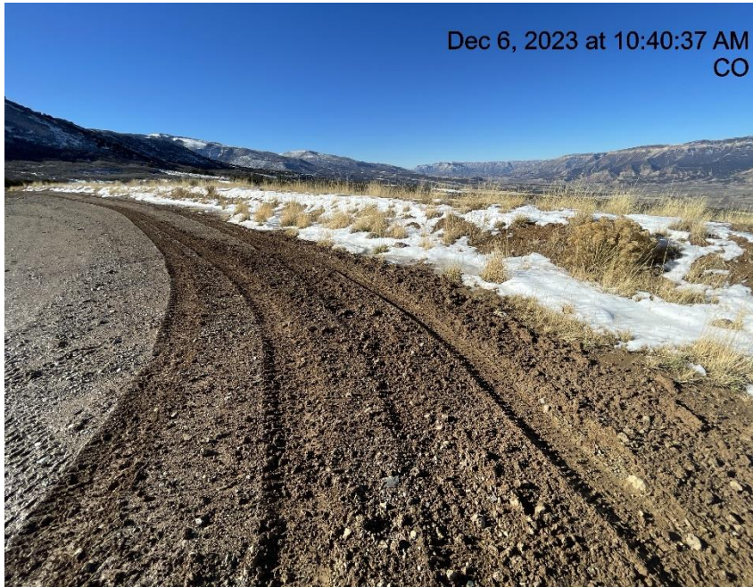
Photo # 8615 Lack of stabilization/compaction/insufficient BMP's
