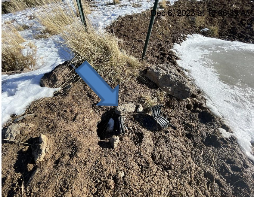
Photo # 8635 Drain needs maintenance
