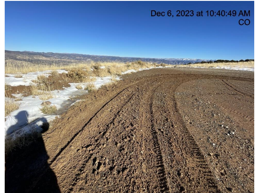
Photo # 8616 Lack of stabilization/compaction/insufficient BMP's
