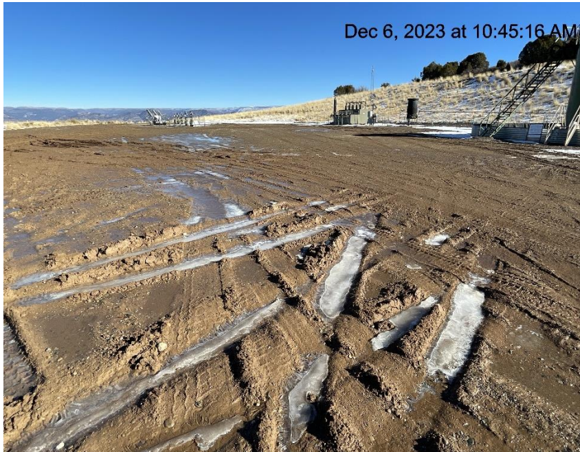
Photo # 8629 Lack of stabilization/compaction/insufficient BMP's
