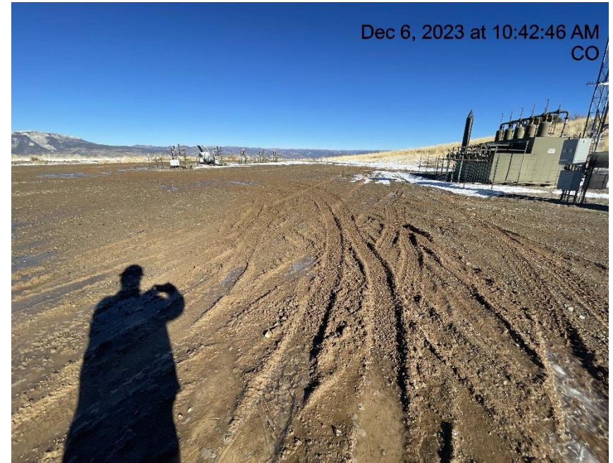
Photo # 8620 Lack of stabilization/compaction/insufficient BMP's
