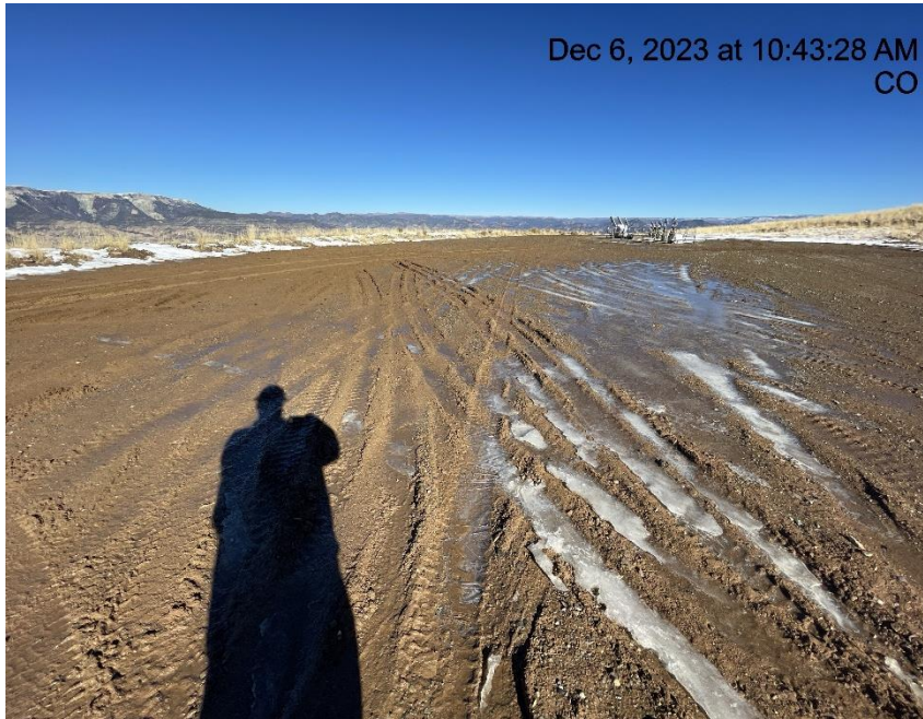
Photo # 8621 Lack of stabilization/compaction/insufficient BMP's
