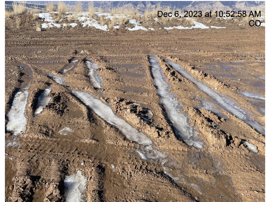
Photo # 8634 Lack of stabilization/compaction/insufficient BMP's
