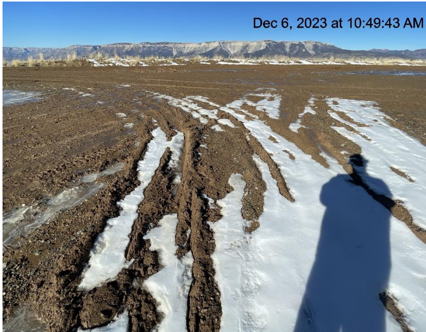
Photo # 8633 Lack of stabilization/compaction/insufficient BMP's
