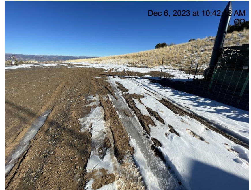
Photo # 8618 Lack of stabilization/compaction/insufficient BMP's
