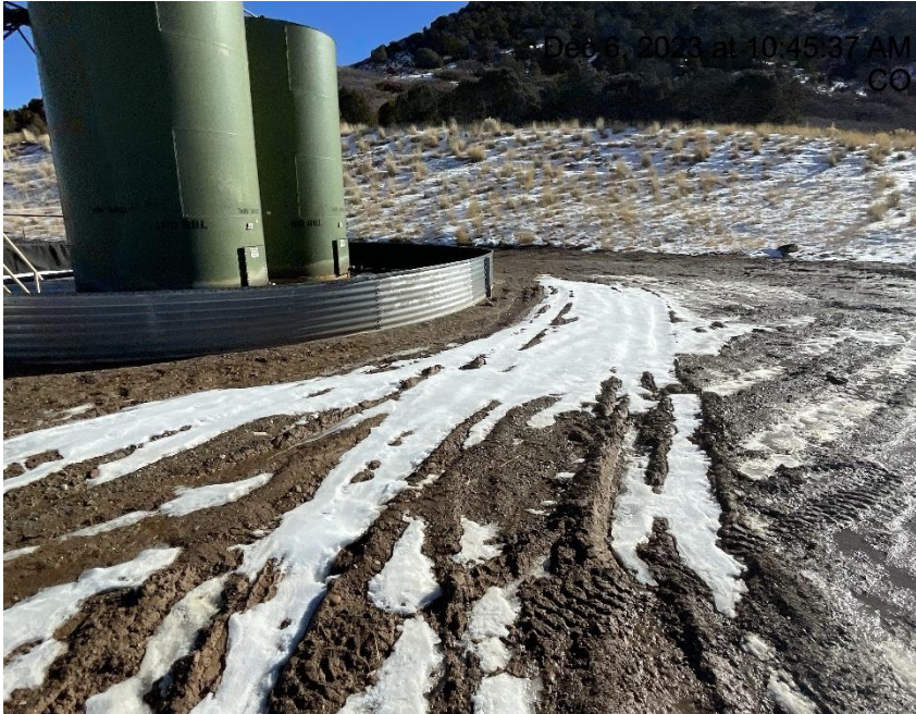
Photo # 8631 Lack of stabilization/compaction/insufficient BMP's
