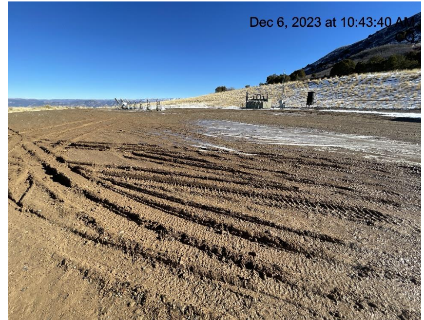
Photo # 8622 Lack of stabilization/compaction/insufficient BMP's
