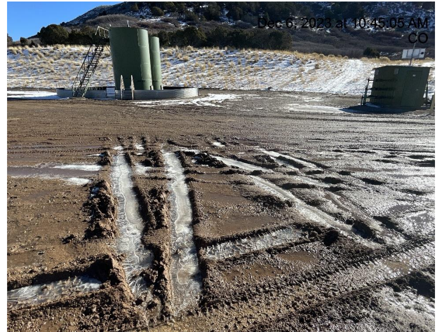
Photo # 8628 Lack of stabilization/compaction/insufficient BMP's
