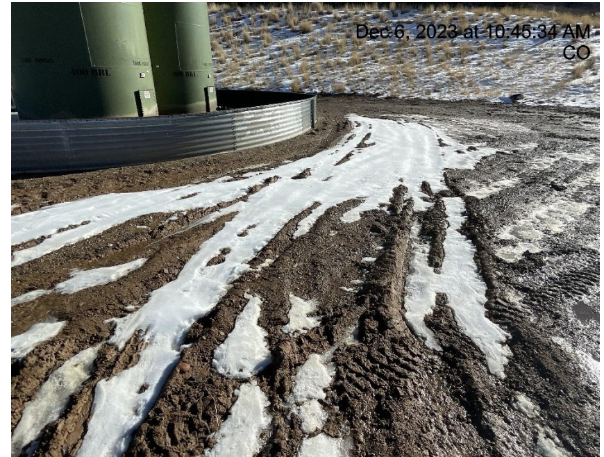
Photo # 8630 Lack of stabilization/compaction/insufficient BMP's
