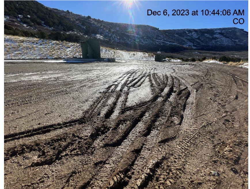
Photo # 8624 Lack of stabilization/compaction/insufficient BMP's
