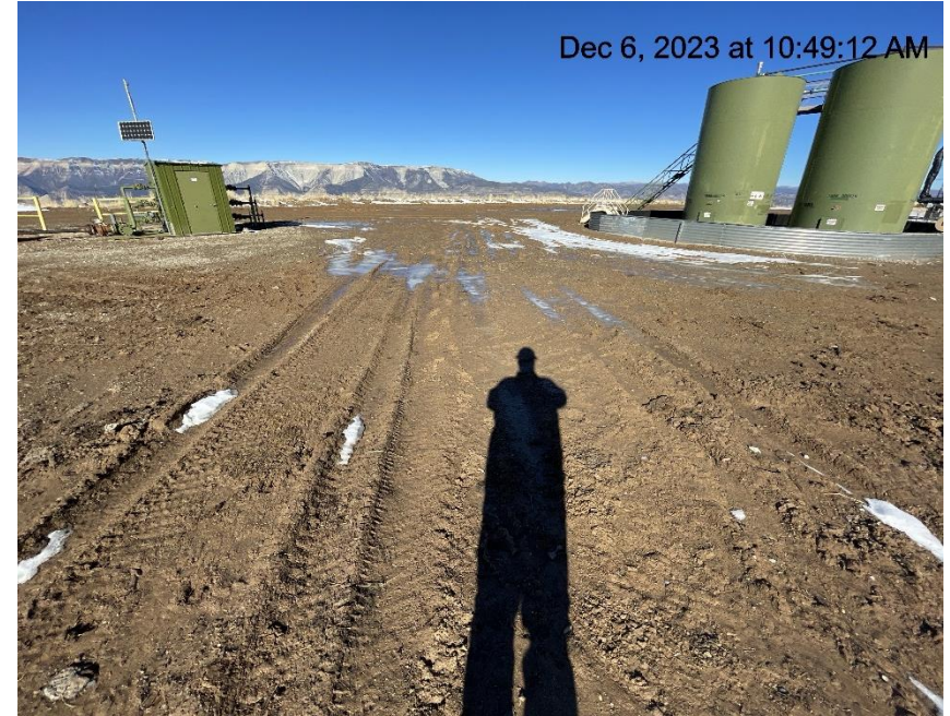
Photo # 8632 Lack of stabilization/compaction/insufficient BMP's
