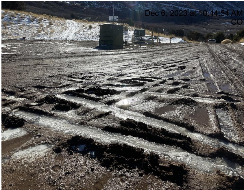
Photo # 8627 Lack of stabilization/compaction/insufficient BMP's
