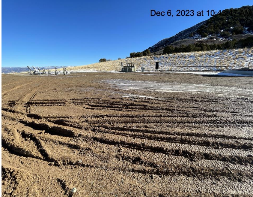
Photo # 8623 Lack of stabilization/compaction/insufficient BMP's
