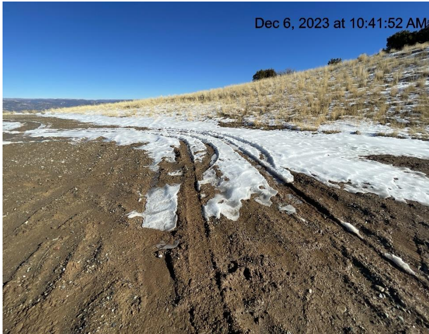
Photo # 8617 Lack of stabilization/compaction/insufficient BMP's
