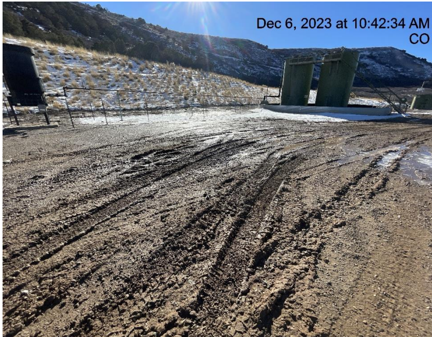
Photo # 8619 Lack of stabilization/compaction/insufficient BMP's
