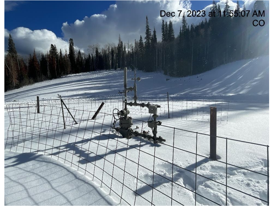
Photo # 8782 Wellhead lacks signage
