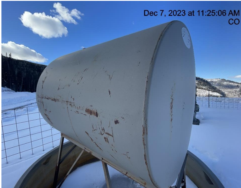
Photo # 8746 Methanol tank improperly labeled/lacks required information (tank near wellhead)
