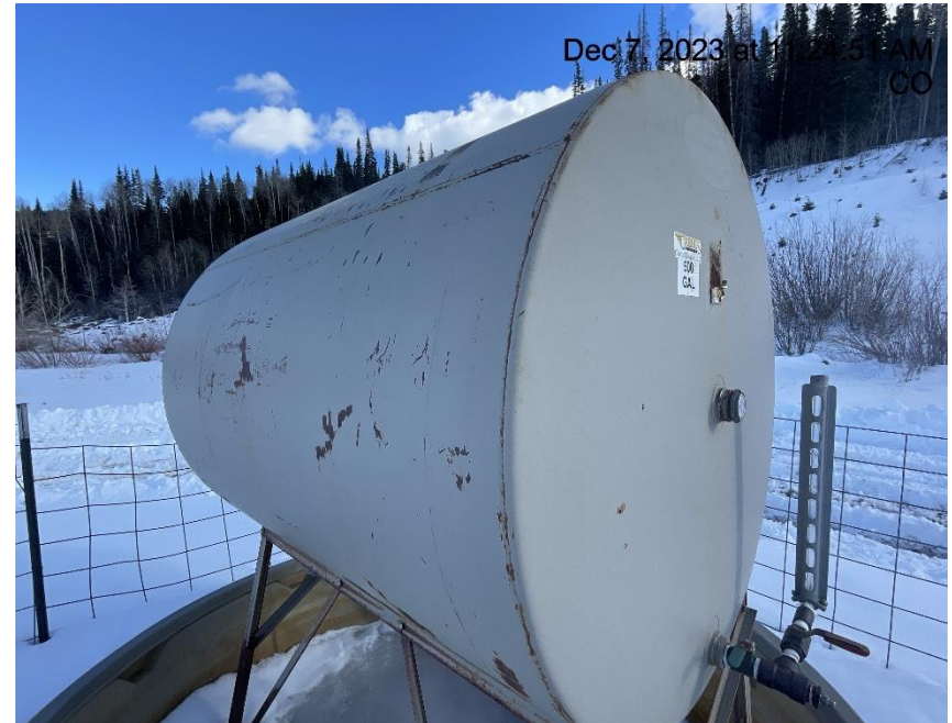
Photo # 8745 Methanol tank improperly labeled/lacks required information (tank near wellhead)
