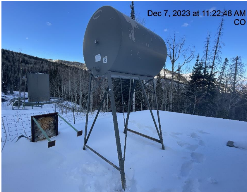
Photo # 8748 Methanol tank lacks secondary containment (tank near separator)
