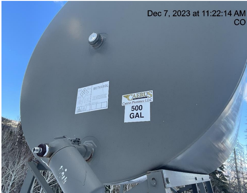
Photo # 8744 Methanol tank label weathered & illegible/improperly labeled/lacks required information (tank near separator)
