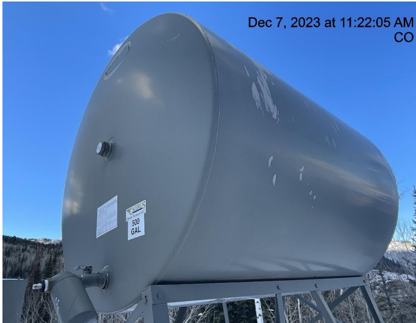
Photo # 8742 Methanol tank label weathered & illegible /improperly labeled/lacks required information (tank near separator)
