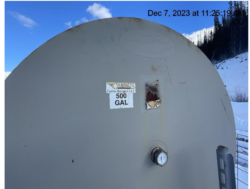
Photo # 8747 Methanol tank improperly labeled/lacks required information (tank near wellhead)
