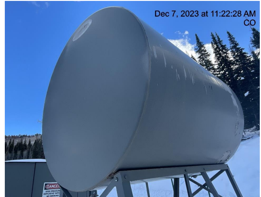
Photo # 8743 Methanol tank improperly labeled/lacks required information (tank near separator)
