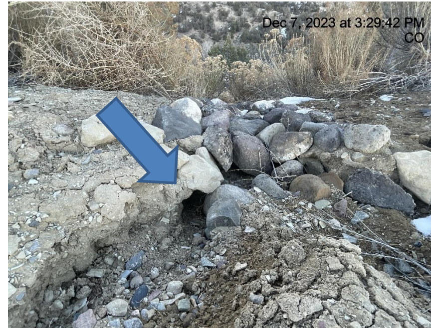
Photo # 8986 Rip Rap Run needs maintenance - stormwater is eroding & undercutting Rip Rap Run
