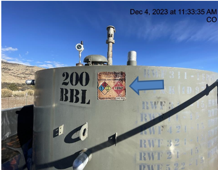
Photo # 8311 Tank label weathered & illegible
