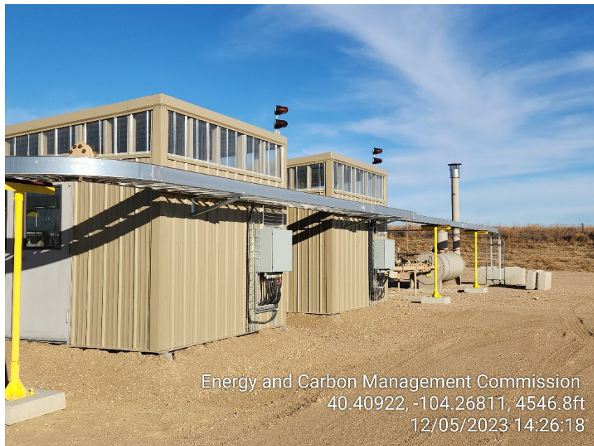
Photo 5 – Gas Lift Injection Meters and Line Heater
