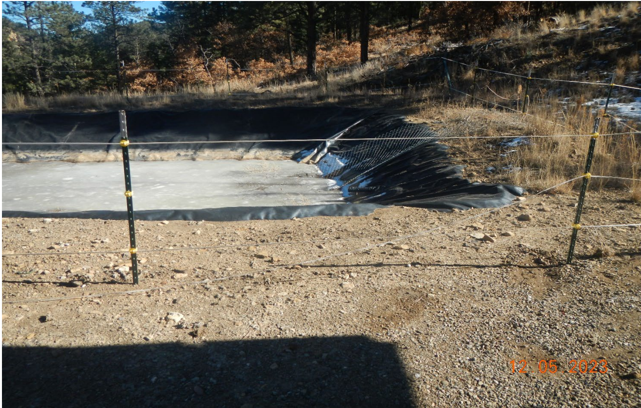
Photo 4. The fence around the lined pi is in disrepair.
