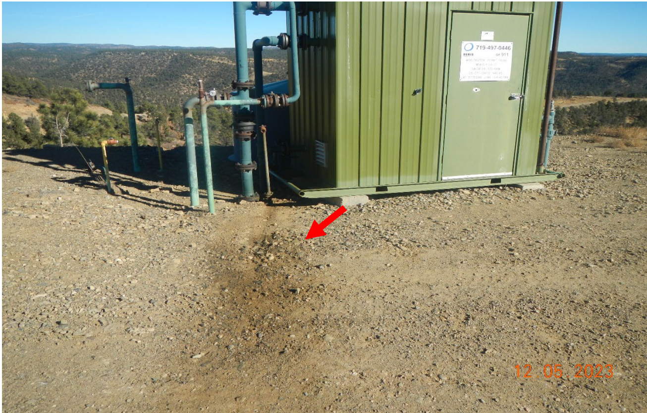
Photo 2. There is stained soil shown at red arrow that needs to be cleaned up. It appears fluids were released at this area.
