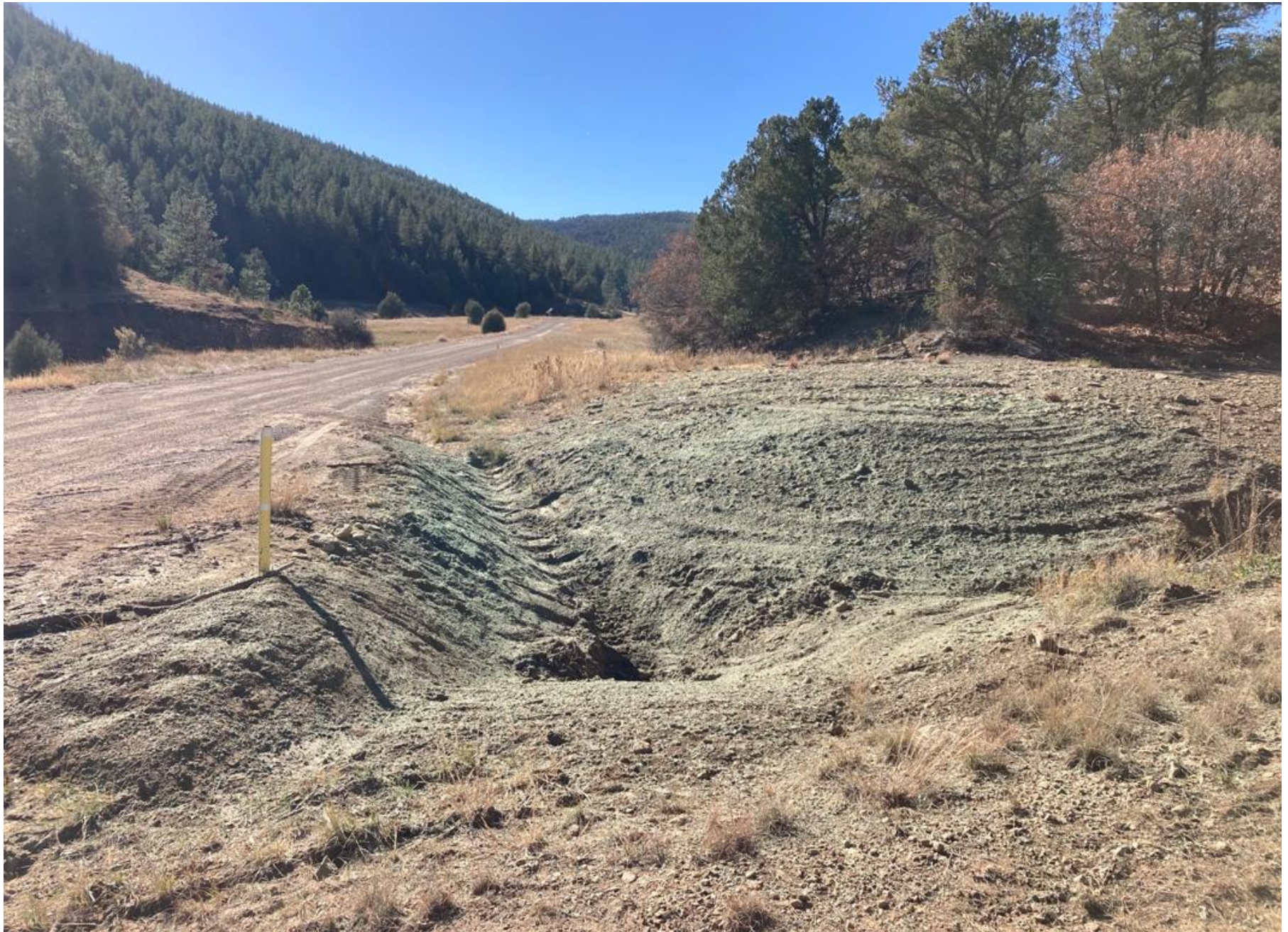
PHOTO 1: THE CULVERT INLET HAS BEEN CLEANED OF SEDIMENT AND RESET. ALL DISTURBED AREAS HAVE BEEN COMPACTED AND SEEDED TO PROMOTE VEGETATIVE STABILIZATION.
