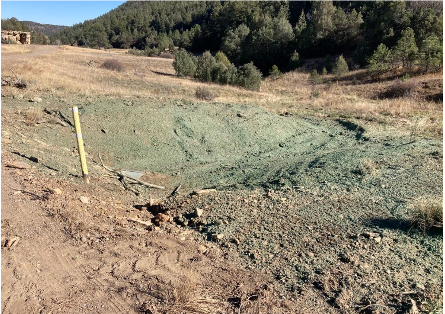
PHOTO 2: THE CULVERT OUTLET HAS BEEN CLEANED OF SEDIMENT AND RESET. ALL DISTURBED AREAS HAVE BEEN COMPACTED AND SEEDED TO PROMOTE VEGETATIVE STABILIZATION. THIS AREA, AND SEVERAL OTHERS ALONG THE MAIN ACCESS, WILL BE FURTHER MONITERED.
