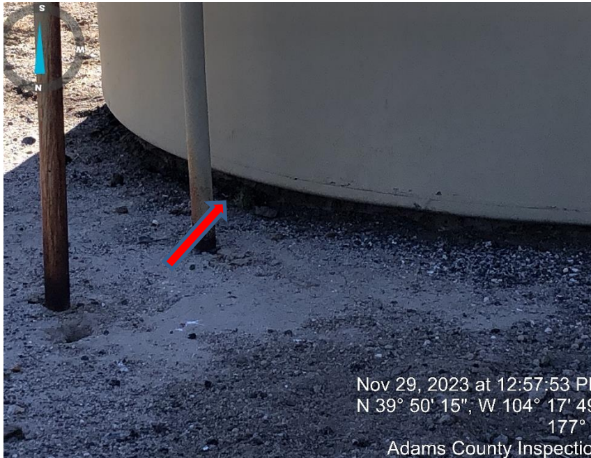
Photo #3 Berm eroded under crude tank.
