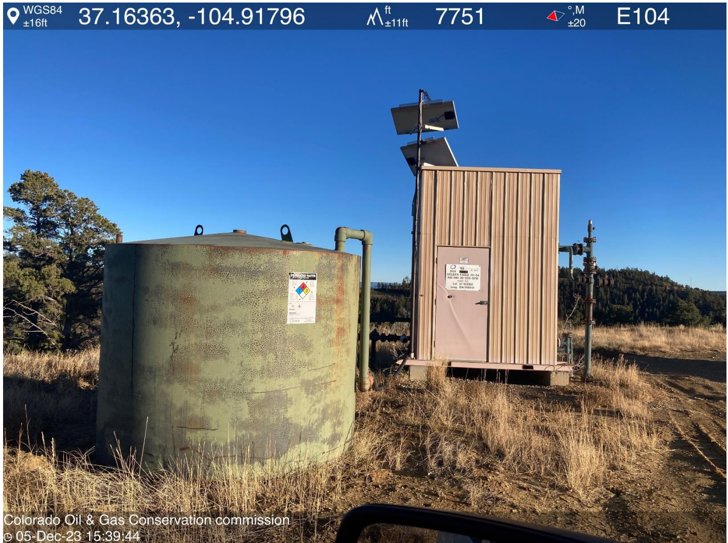
PHOTO 4: PRODUCED WATER TANK.
