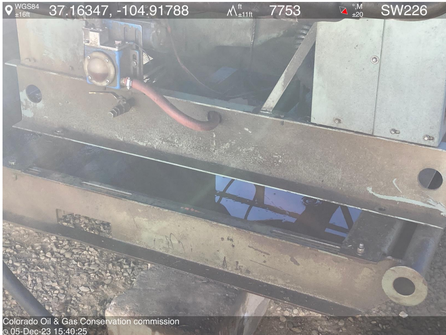
PHOTO 6: OILY WASTE IN ENGINE SKID. COMPLY WITH RULE 1002.f.(2)B, Comply with general provisions of the oil and gas act for wildlife protection AND SB-181. CA DATE 12-6-2023.
