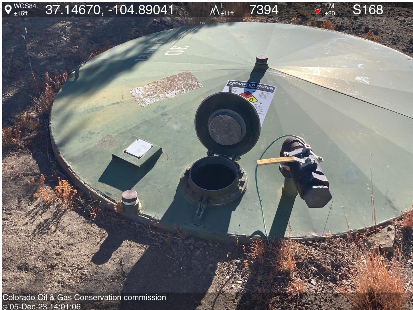
PHOTO 6: GAUGE HATCH IS OPEN. Close and seal gauge hatches when not accessing tank per Rule 608.a.(9). CA DATE 12-6-2023.
