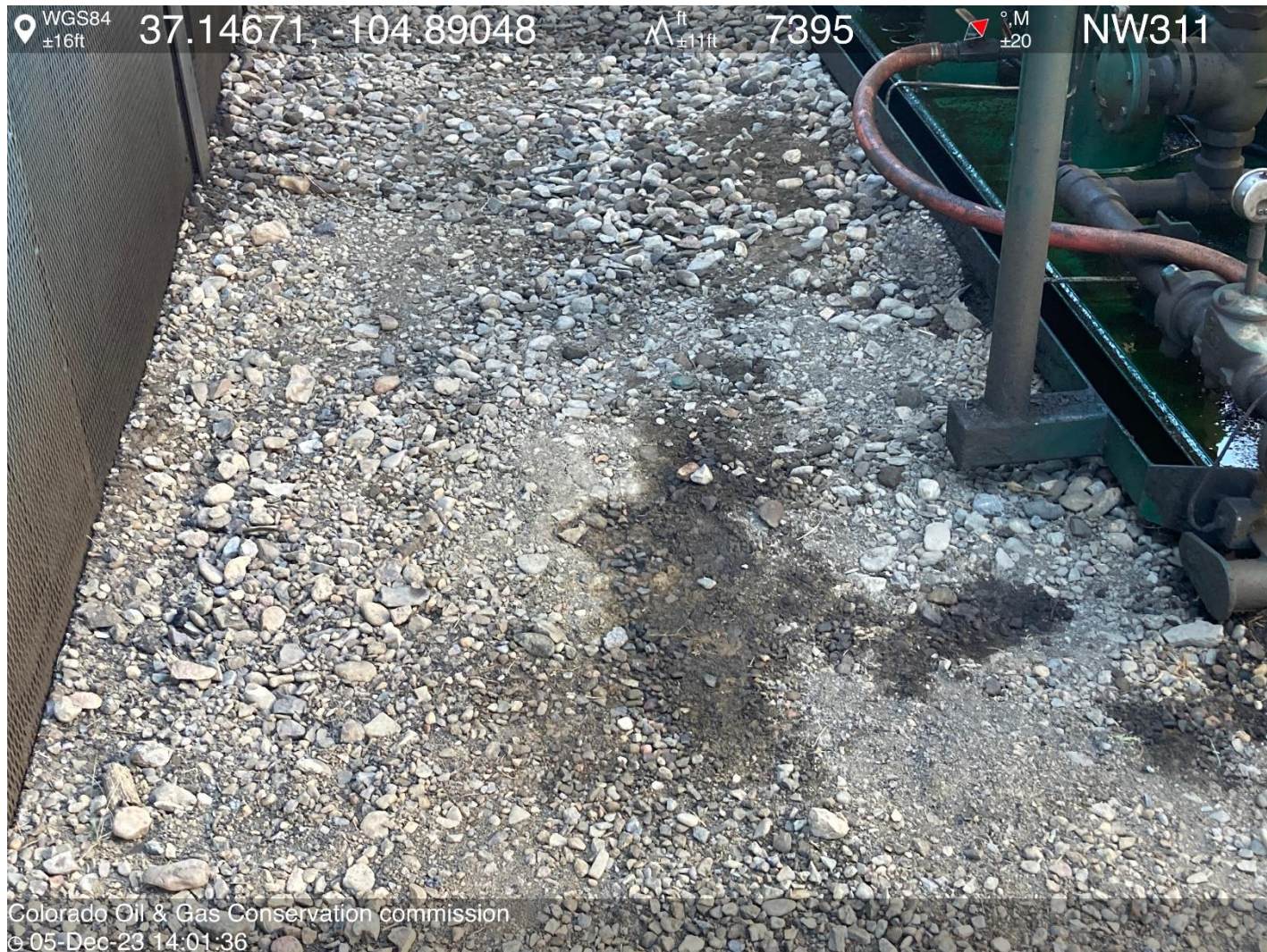
PHOTO 5: AREA OF IMPACTED SOIL NEAR COMPRESSOR FOR ORIGINAL WELL. Conduct maintenance on equipment, cleanup stained material and review self inspection processes. COMPLY WITH RULE 1002,.(2).D. CA DATE 01-5-2024.
