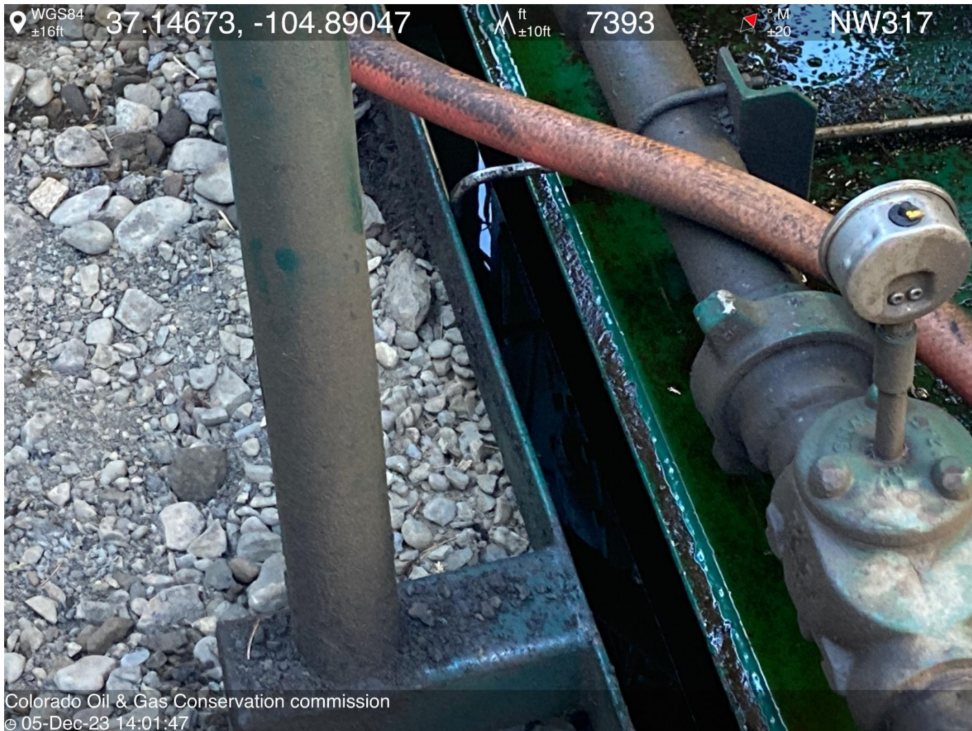
PHOTO 7: OILY WASTE IN ENGINE SKID. COMPLY WITH RULE 1002.f.(2)B, Comply with general provisions of the oil and gas act for wildlife protection AND SB-181. CA DATE 12-6-2023.
