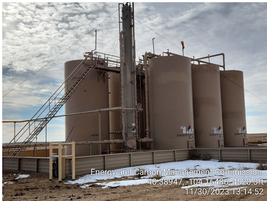
Photo 5 – Tank Battery
