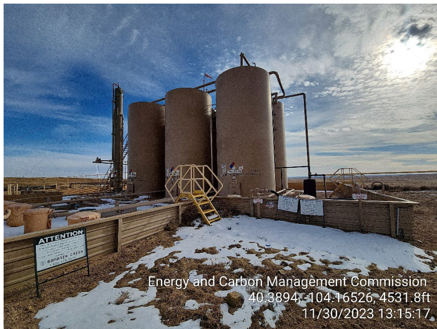
Photo 7 – Tank Battery
