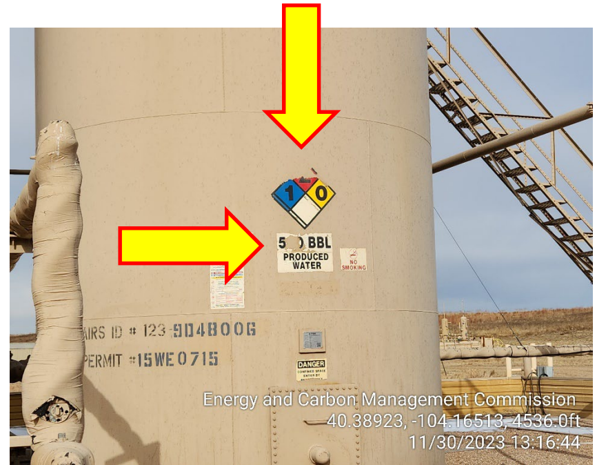
Photo 10 – Water Tank NFPA and Capacity Labels
