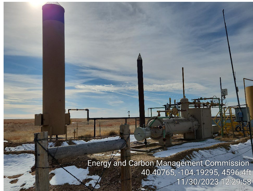
Photo 6 – Separator and ECD
