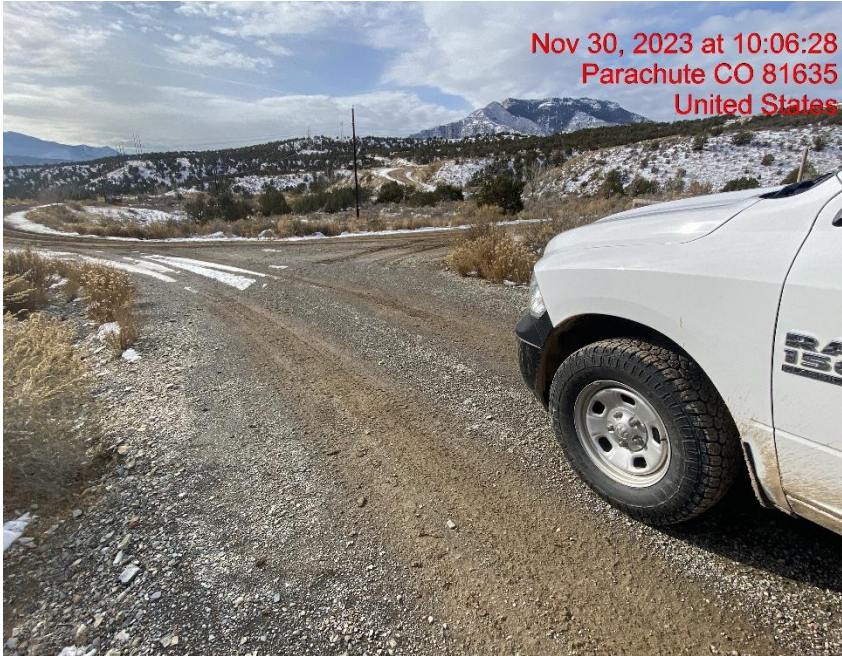
Insufficient Vehicle Tracking BMPs at Location Entrance/Exit – Photo #07773
