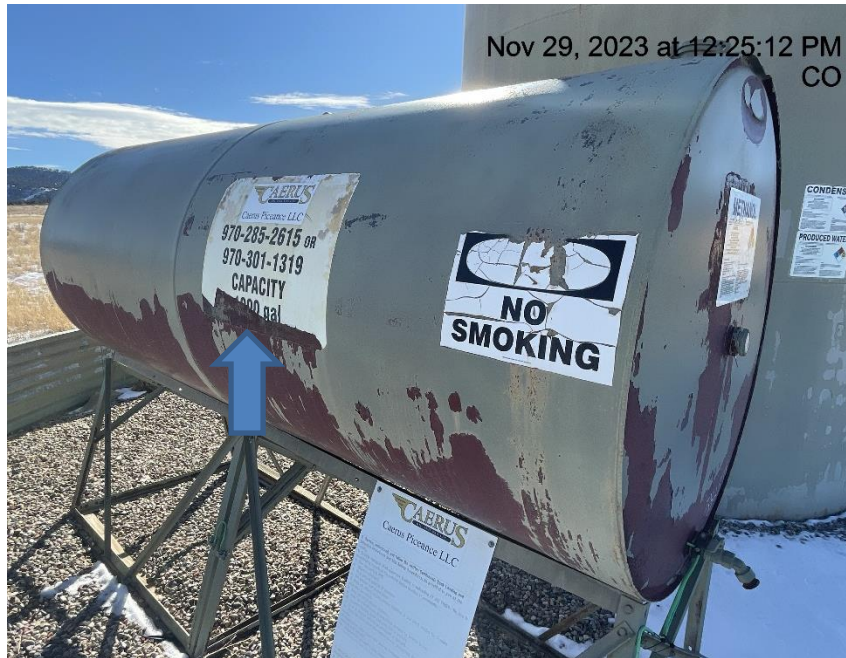
Photo # 7876 Methanol tank label damaged/some info illegible
