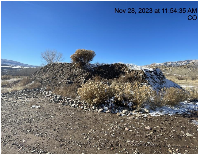
Photo # 7764 Stockpiled soils on location/insufficient BMP's
