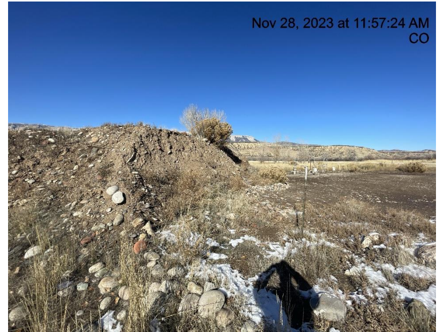
Photo # 7765 Stockpiled soils on location/insufficient BMP's
