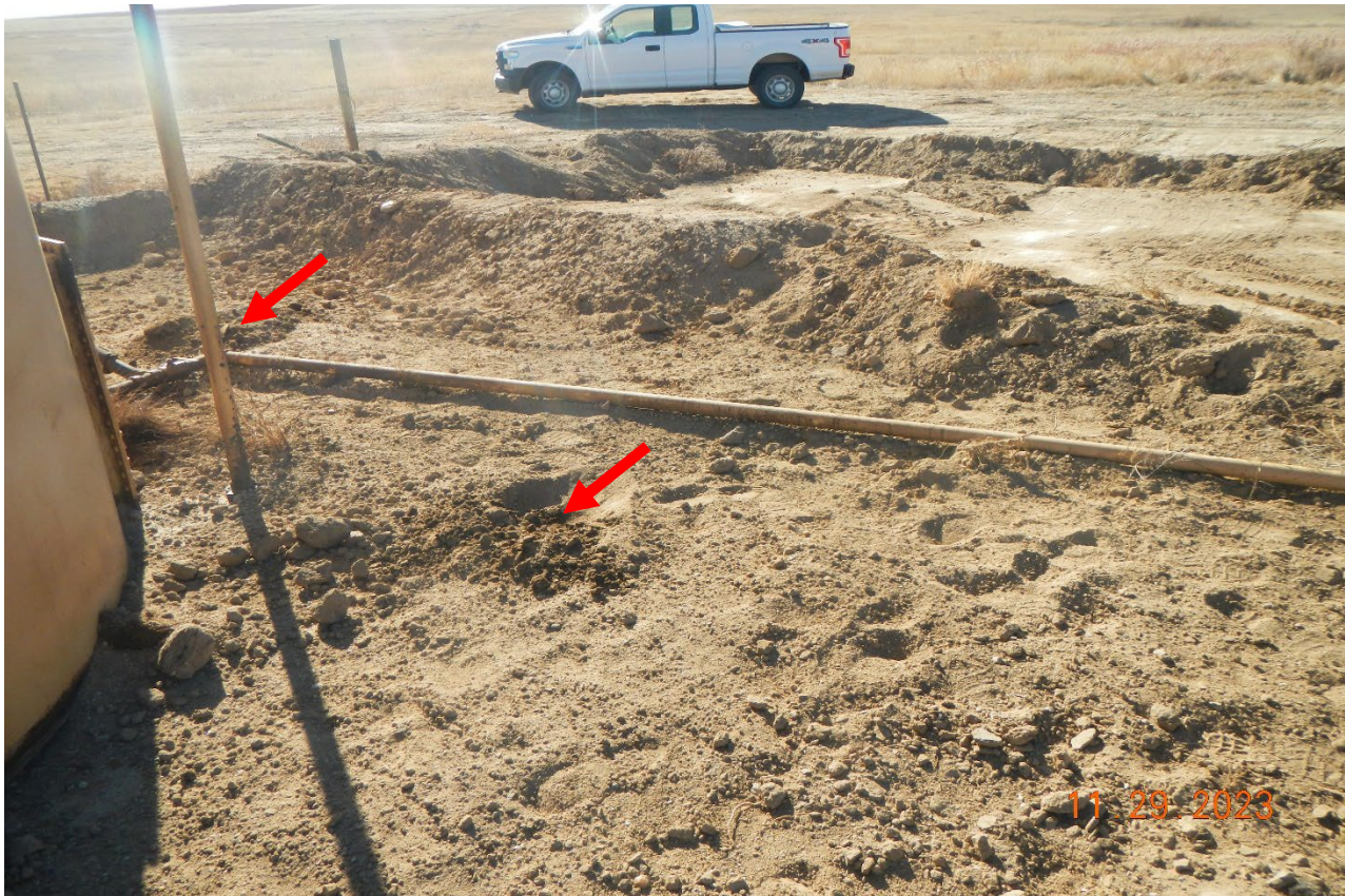
Photo 13. Facing back at the spill area where fresh dirt was spread over the spilled area of oil stained soils. Red arrows show the stained soils that uncovered the dirt laced over the spill area.
