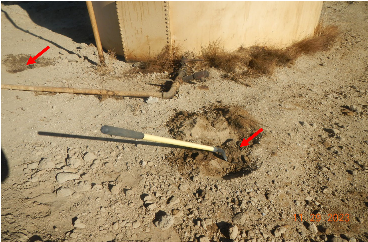
Photo 11. It appears dirt was pushed over the spill area which was not cleaned up. Shovel uncovered the fresh dirt placed over the oil stained soils show the stained oily soils at red arrow.
