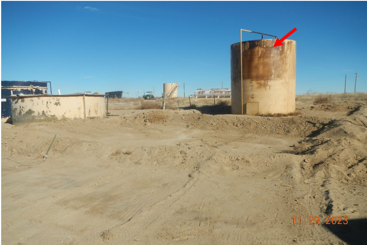
Photo 9. Facing northwest toward the tank battery. There was a recent spill that had occurred at the tank shown at red arrow. Soils have been pushed and secondary containment is not adequate. Loose soils are susceptible to erosion and all contaminated soils need to be cleaned up and removed.
