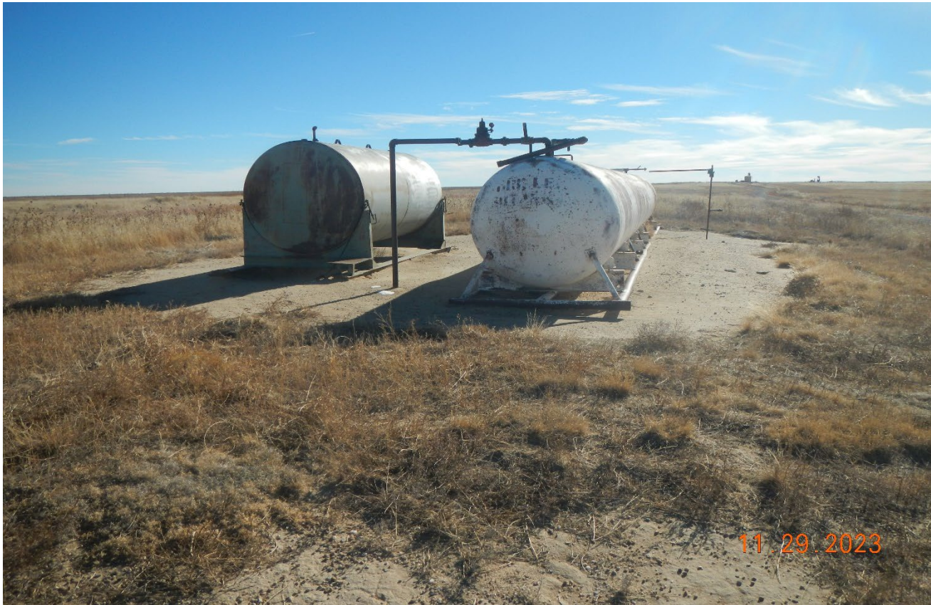
Photo 3. Facing southeast at the location. The two large volume tanks do not have proper labeling or secondary containment. If the tanks are unused then they need to be removed. Previous corrective action was not completed.
