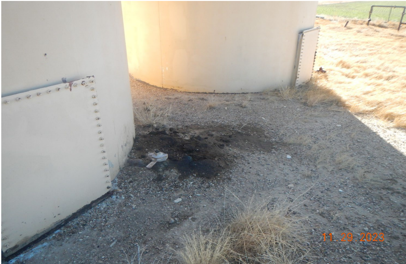
Photo 4. There is oil stained soil at the back side of the tank that needs to be cleaned up.
