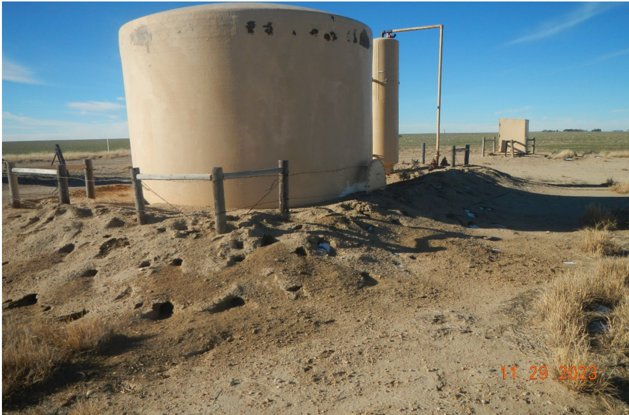
Photo 6. Facing toward the tank. The berm around the tank is inadequate to contain a spill. The fence around the tank is in disrepair. Previous corrective action was not completed.
