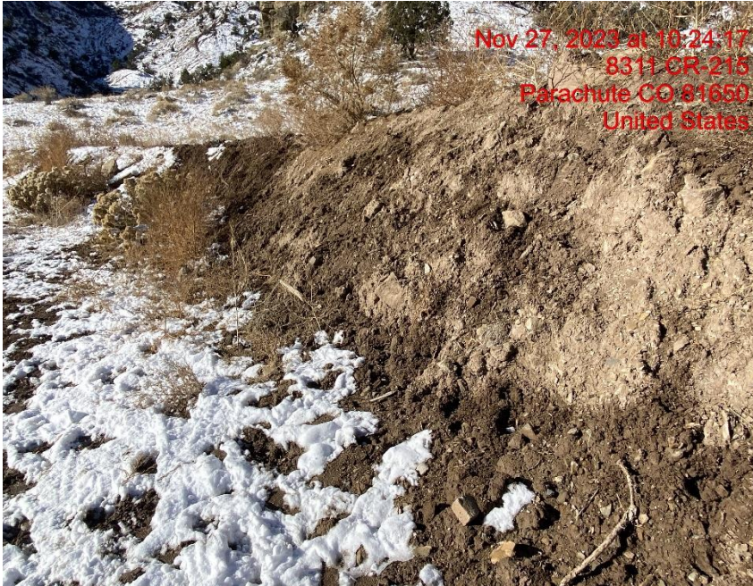
Insufficient Cut Slope Erosion Controls – Photo #07671
