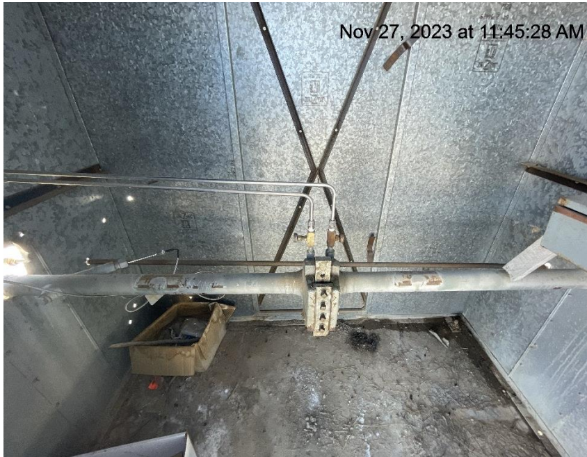
Photo # 7600 No cal card/meter calibration info not conspicuously posted
