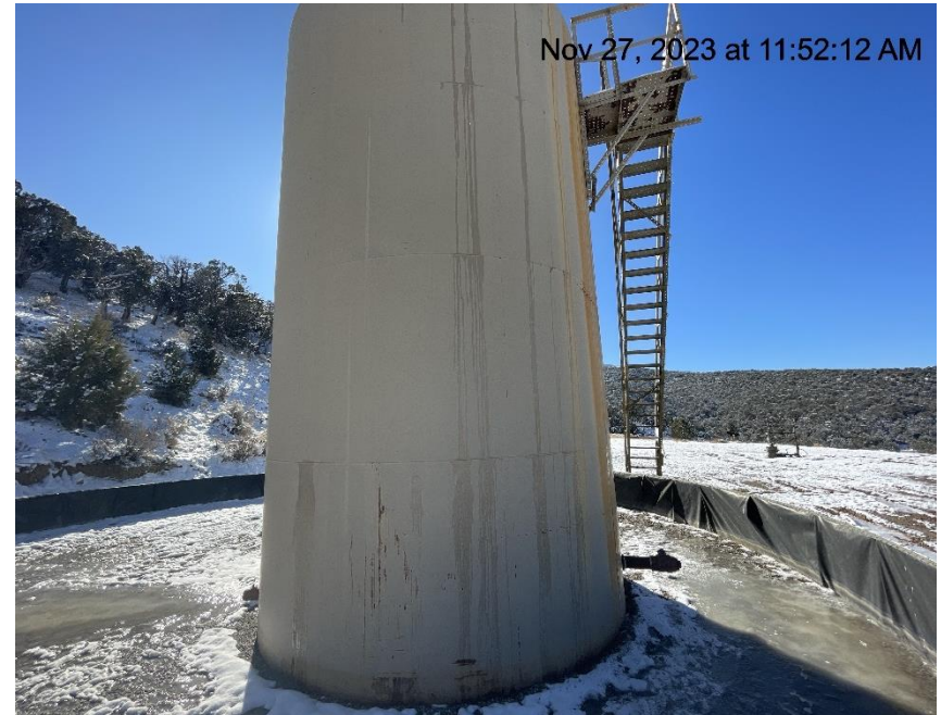
Photo # 7605 Production tank not properly labeled/missing required information
