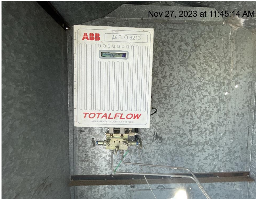
Photo # 7598 No cal card/meter calibration info not conspicuously posted
