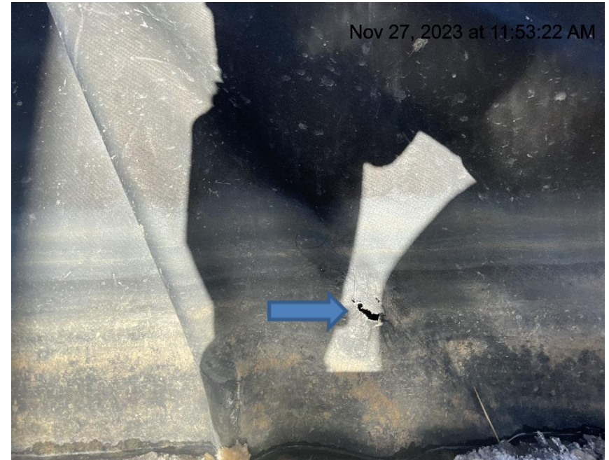
Photo # 7603 Hole in liner/liner needs maintenance
