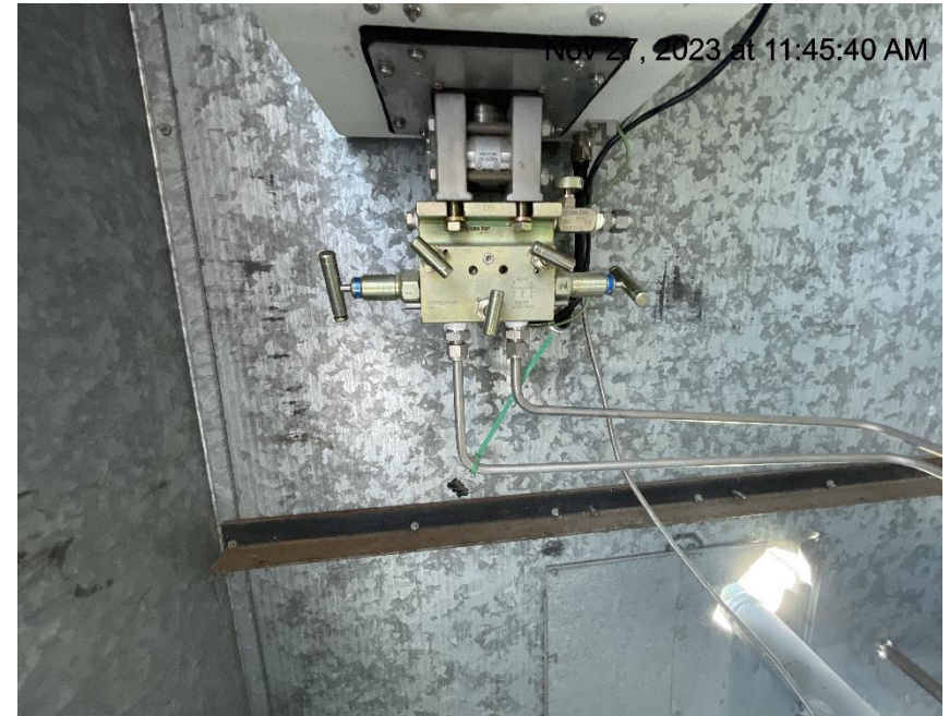
Photo # 7599 No cal card/meter calibration info not conspicuously posted
