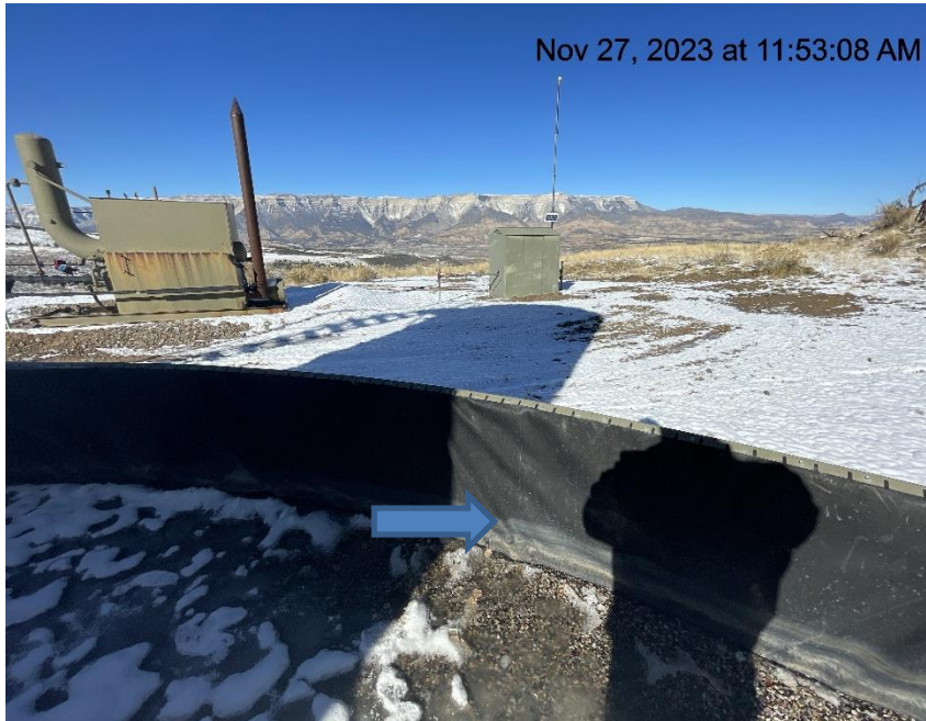
Photo # 7602 Hole in liner/liner needs maintenance
