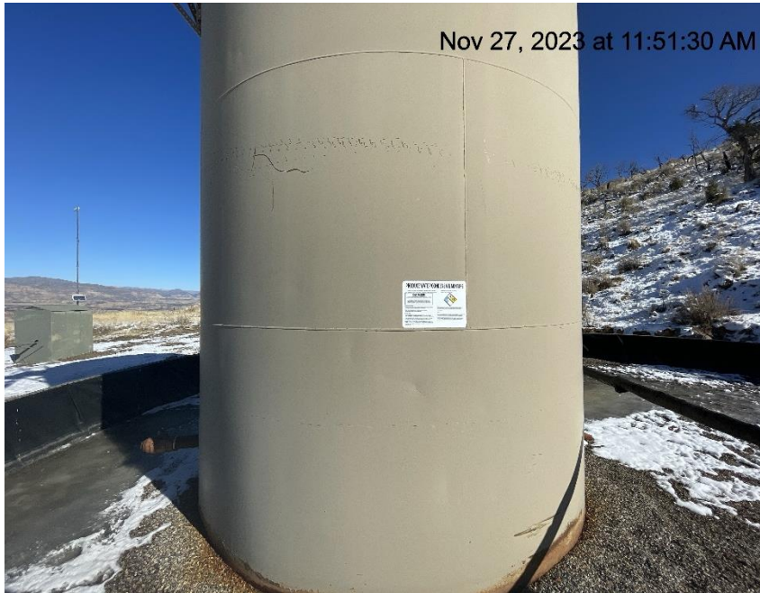
Photo # 7604 Production tank not properly labeled/missing required information
