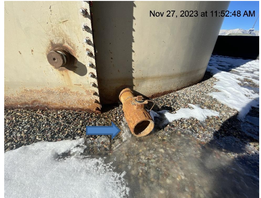
Photo # 7601 Open ended load line
