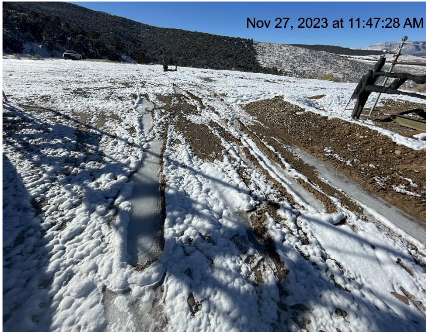
Photo # 7608 Lack of stabilization/compaction
