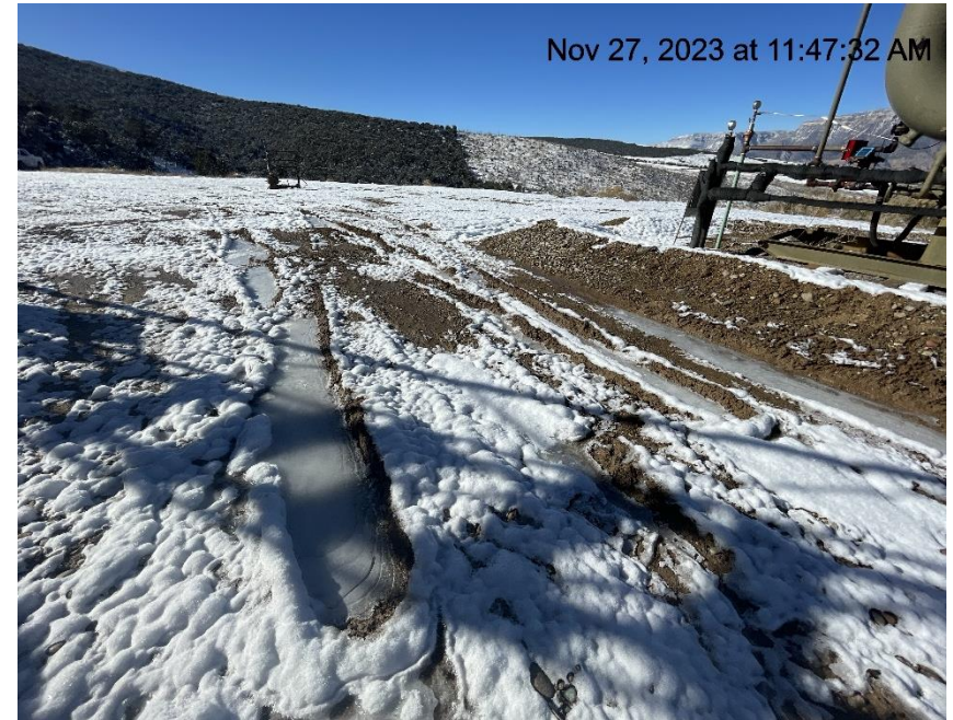
Photo # 7609 Lack of stabilization/compaction
