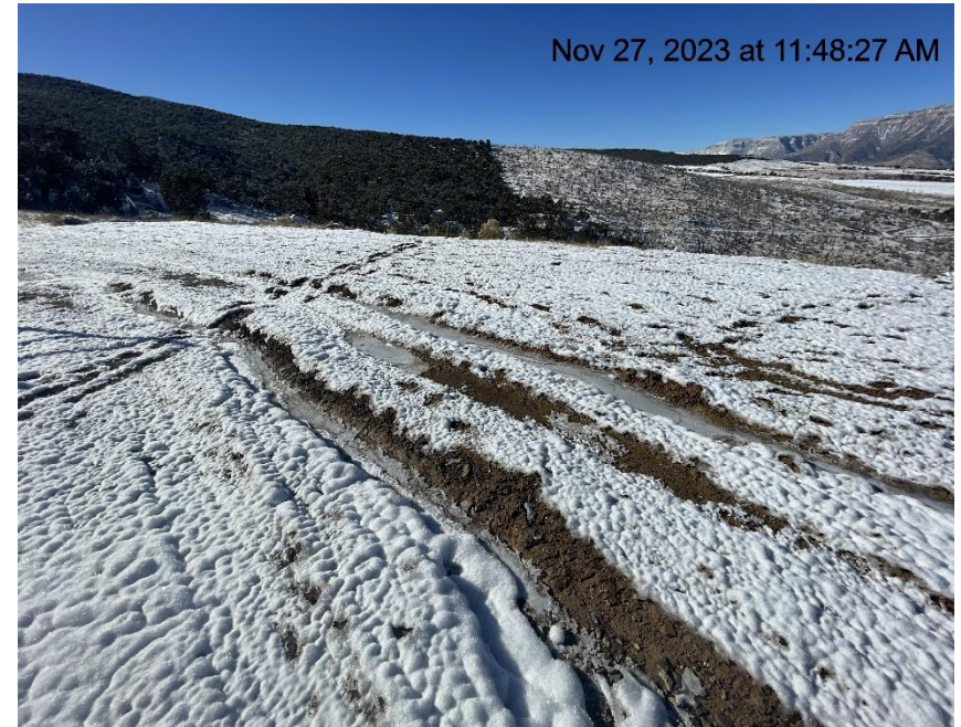
Photo # 7613 Lack of stabilization/compaction
