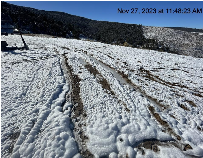
Photo # 7612 Lack of stabilization/compaction
