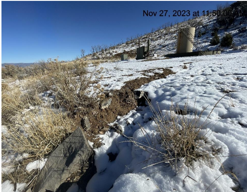
Photo # 7620 Erosion & transport of sediment off location
