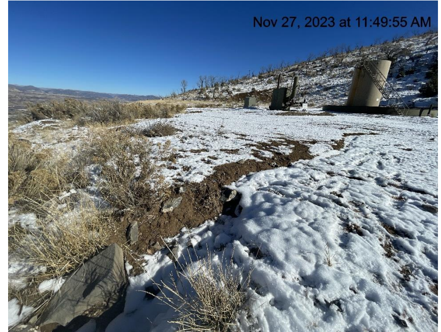
Photo # 7619 Erosion & transport of sediment off location
