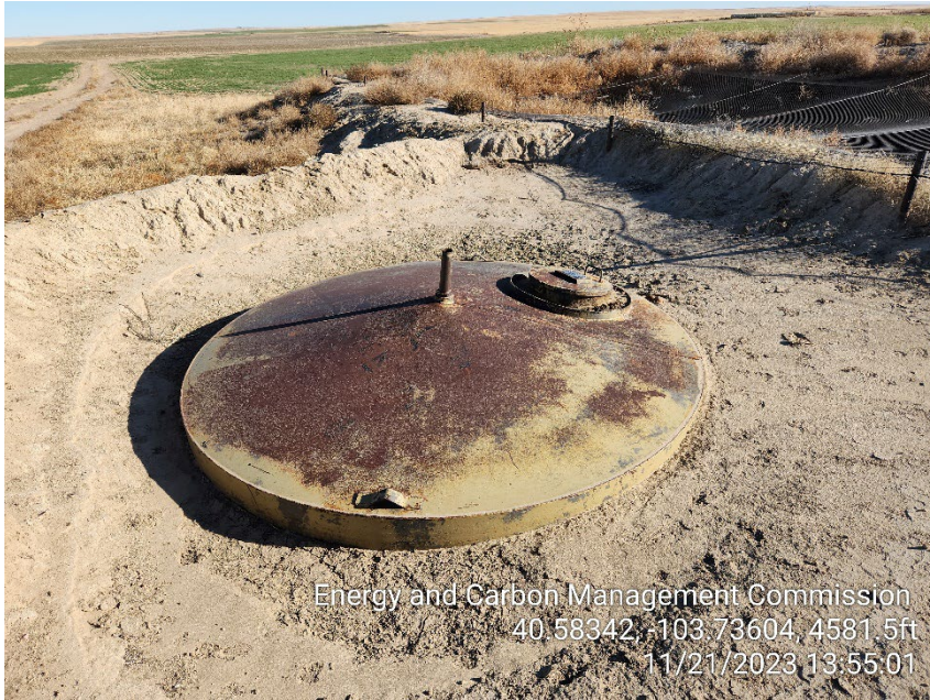
Photo 1 – Skim Tank – NFPA Label missing
