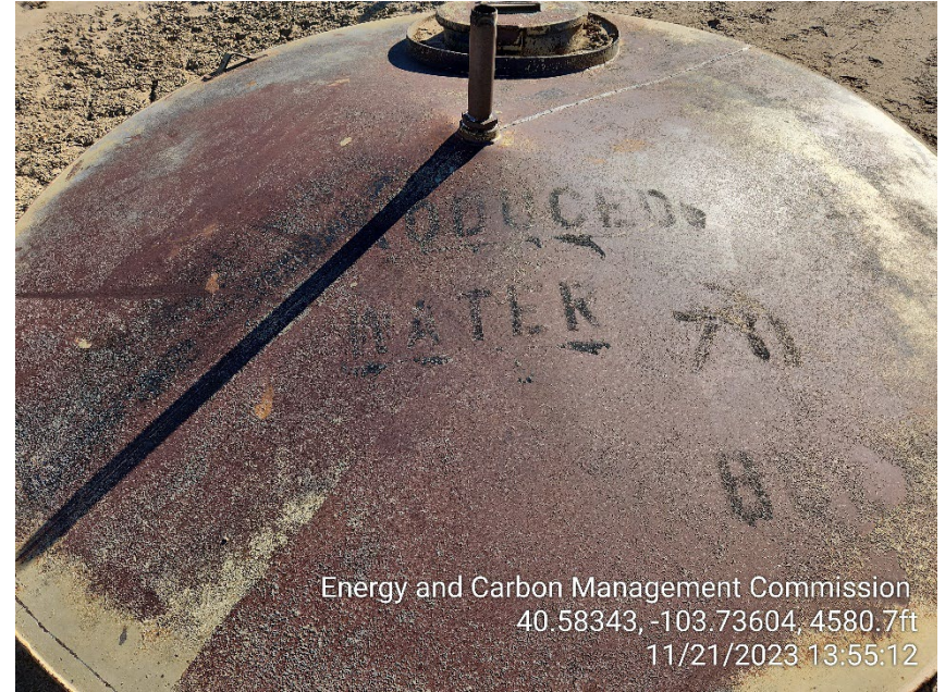
Photo 2 – Skim Tank – NFPA Label missing
