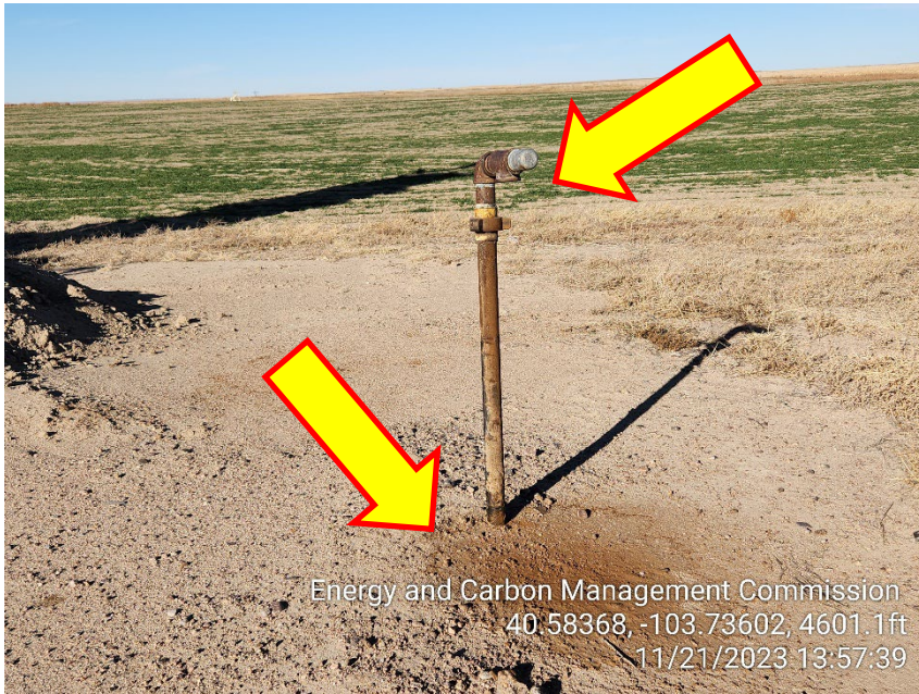
Photo 13 – Riser East of Heater Treater not marked with OOSLAT and Stained Soil
