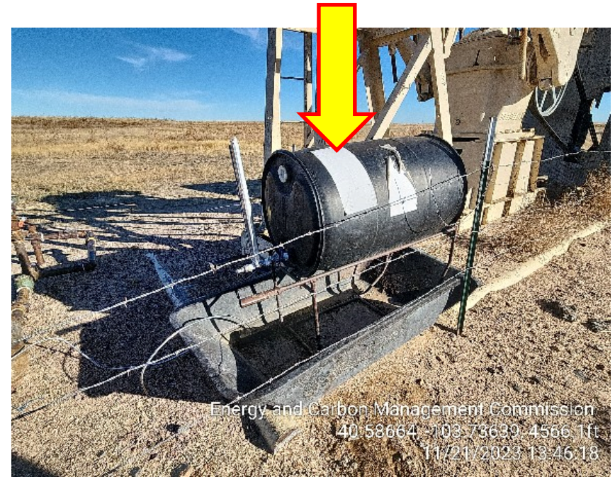
Photo 4 – Chemical Tank – Label has faded no longer visible
