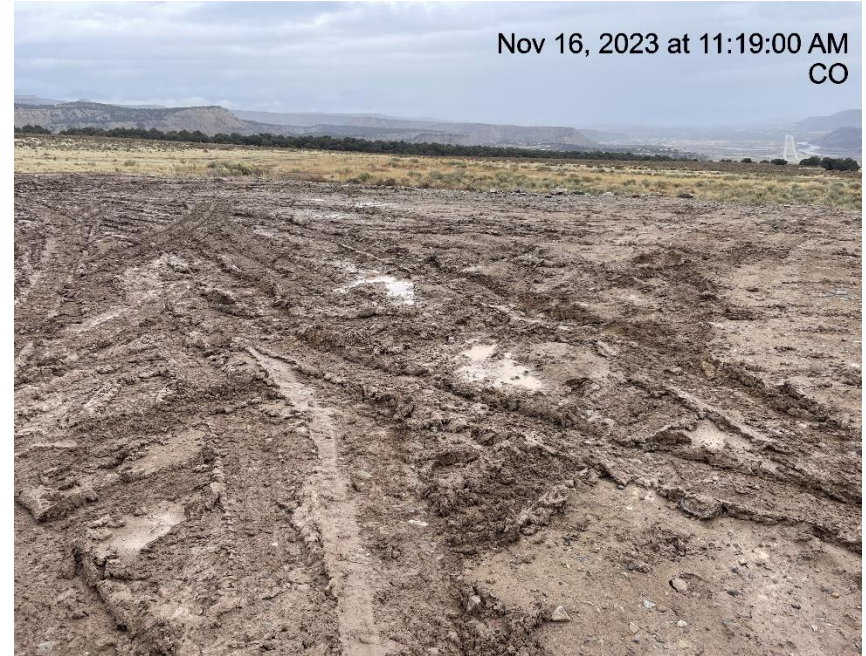
Photo # 6842 Lack of stabilization/compaction
