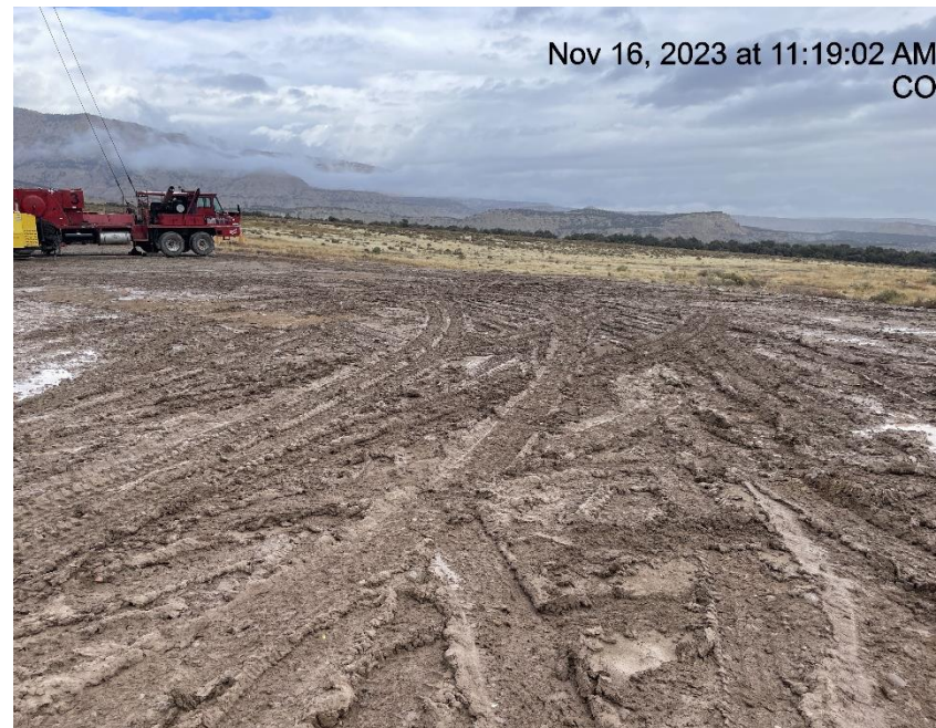
Photo # 6843 Lack of stabilization/compaction
