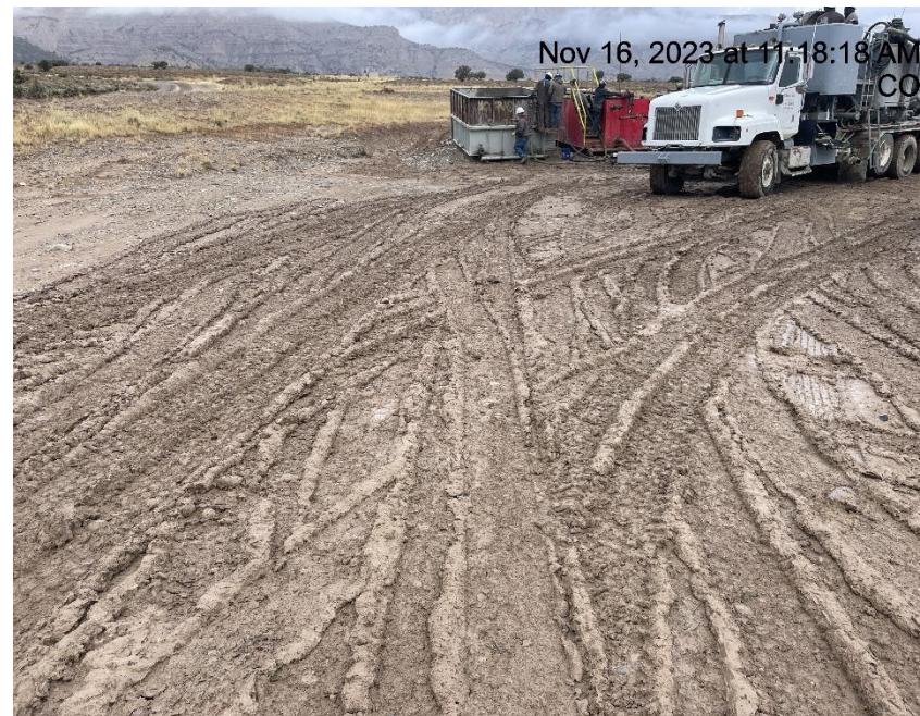
Photo # 6841 Lack of stabilization/compaction
