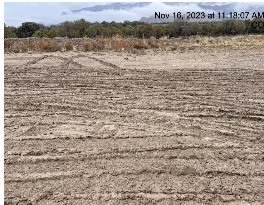
Photo # 6840 Lack of stabilization/compaction
