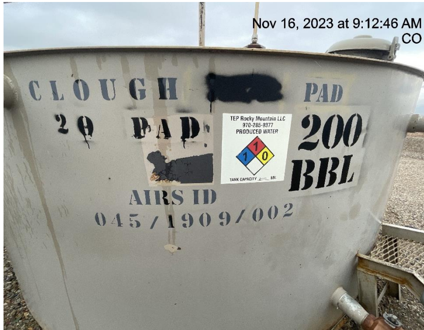
Photo # 6837 Tank capacity incorrect
