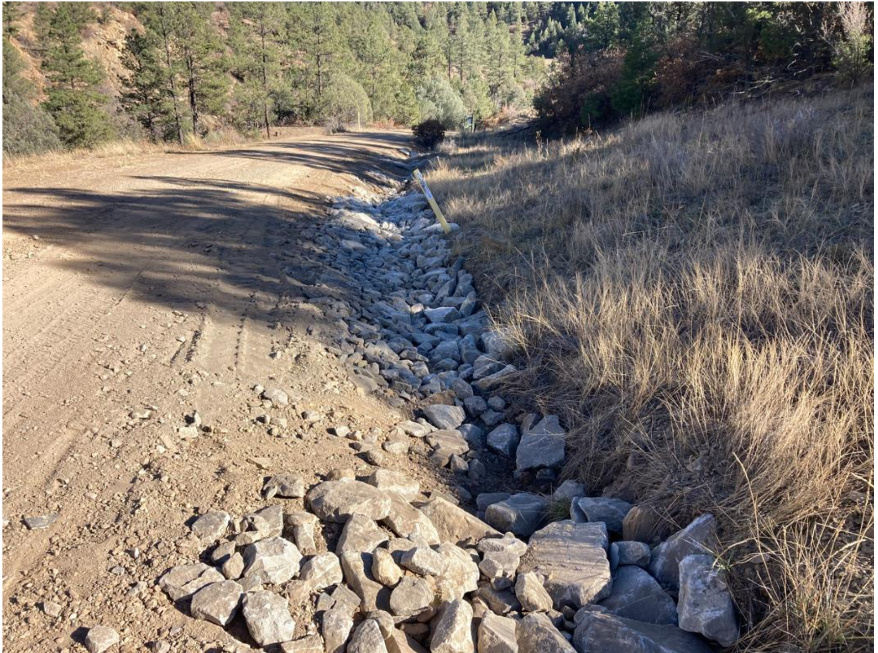
PHOTO 1: THE ENTIRE ACCESS LEADING TO AND PAST THE NEW ELK 25-01 HAS BEEN BLADED, DIVERSION DITCHES REDEFINED, ROCK ADDED WHERE NEEDED, AND CULVERT INLETS/OUTLETS CLEANED AND RESET.THE UNUSED HYDRAULIC HOSES ON LOCATION HAVE ALSO BEEN REMOVED.
