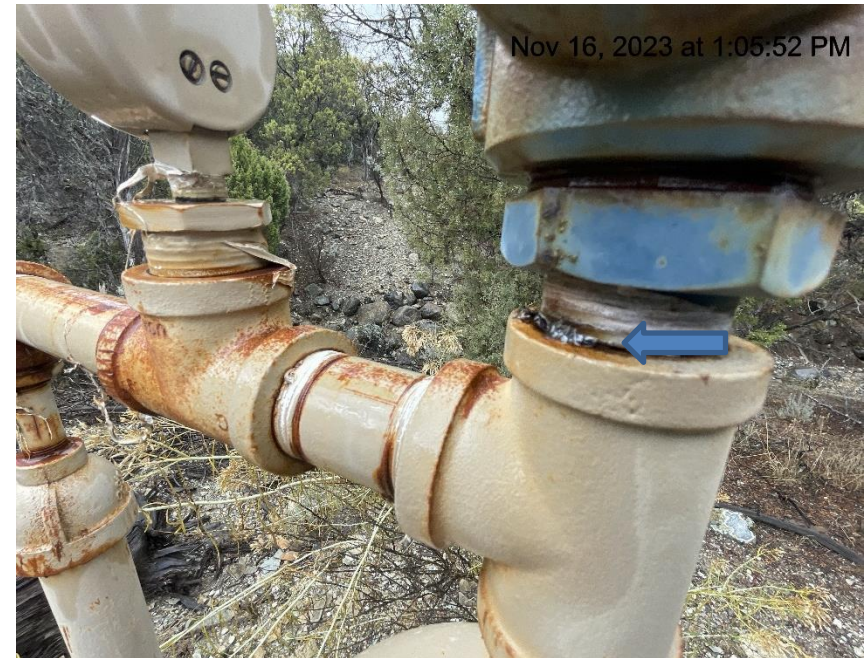
Photo # 6988 Possible leak on PRV
