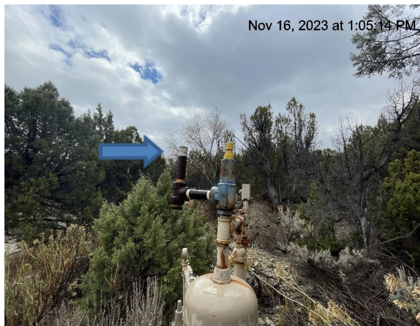
Photo # 6985 PRV vent line lacks cap
