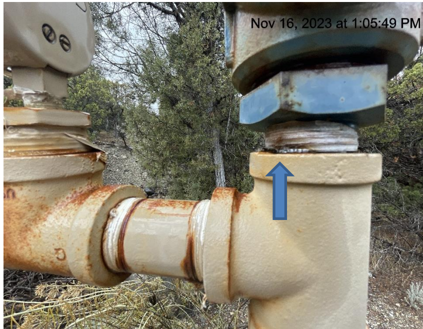
Photo # 6987 Possible leak on PRV
