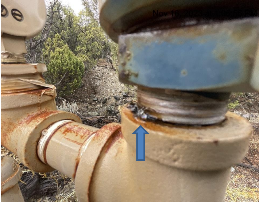
Photo # 6989 Possible leak on PRV
