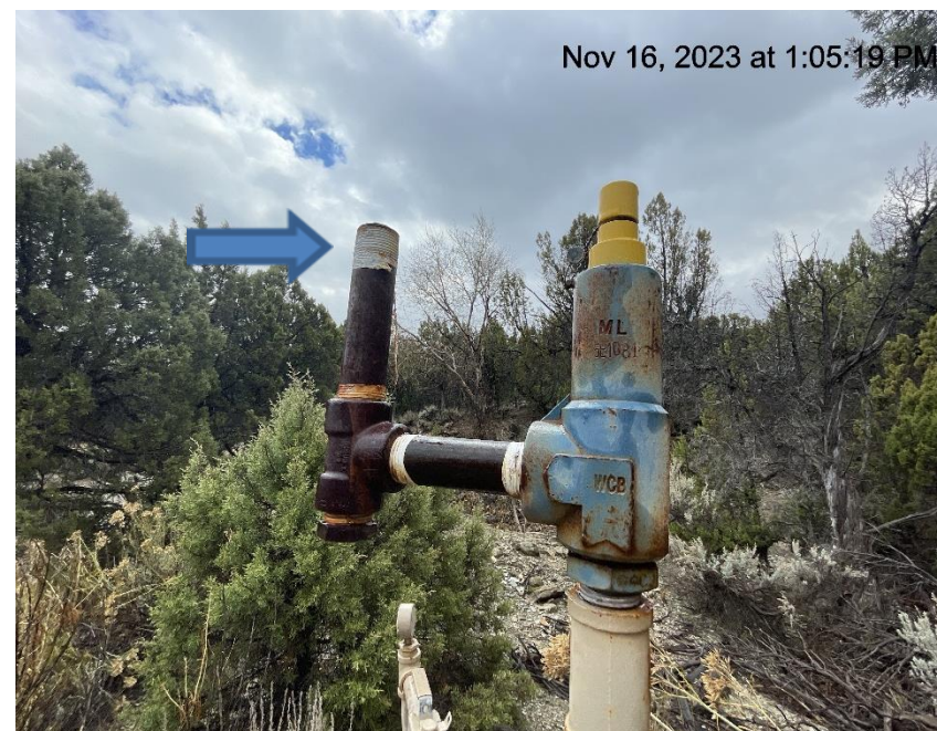
Photo # 6986 PRV vent line lacks cap
