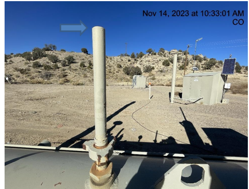
Photo # 6483 Rupture disc vent line lacks cap
