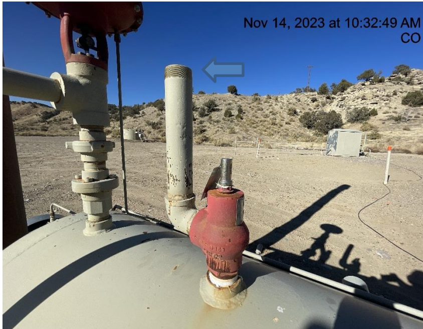
Photo # 6484 PRV vent line lacks cap
