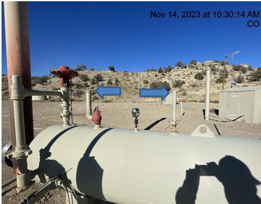
Photo # 6482 PRV & rupture disc vent lines lack caps
