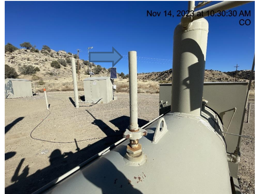
Photo # 6485 Observed distortion coming off rupture disc vent line/rupture disc leaking gas
