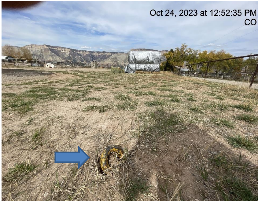
Photo # 4059 From inspection 708902036 conducted on 10/24/2023 Unmarked deadman
